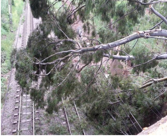
Figure 1: Trees falling on OHE
