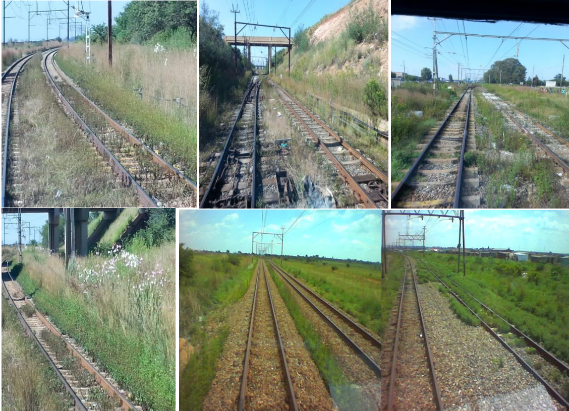
Figure 5: Overgrown vegetation on railway tracks.
