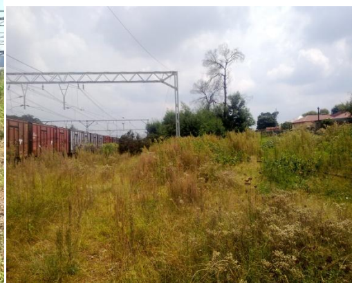
Figure 4: Vegetation poses fire hazard
