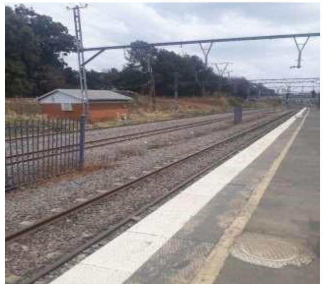
Picture 4: Vandalised fencing at the station
