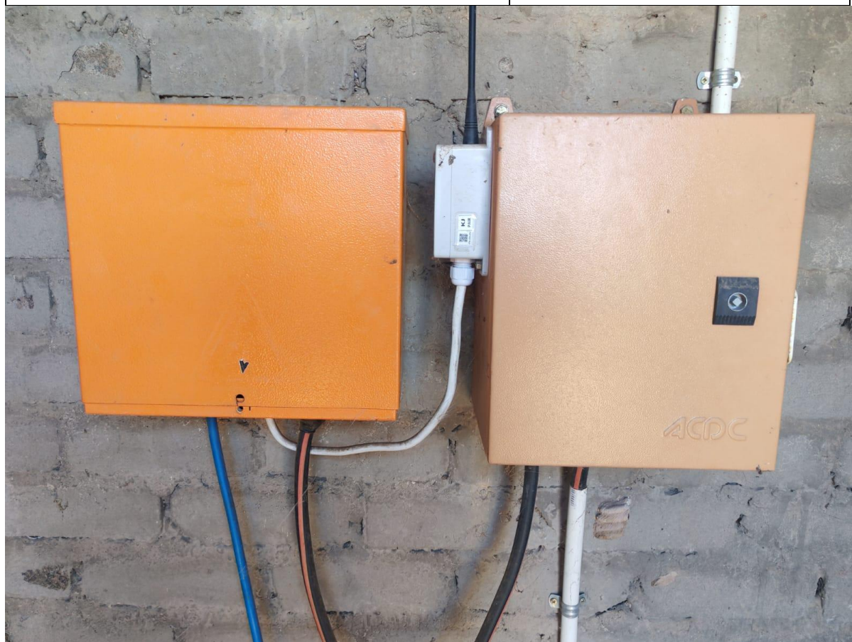
Figure 3 Pump Control Box and DB for Submersible Pump (The current power source is to be replaced by solar PV system)
