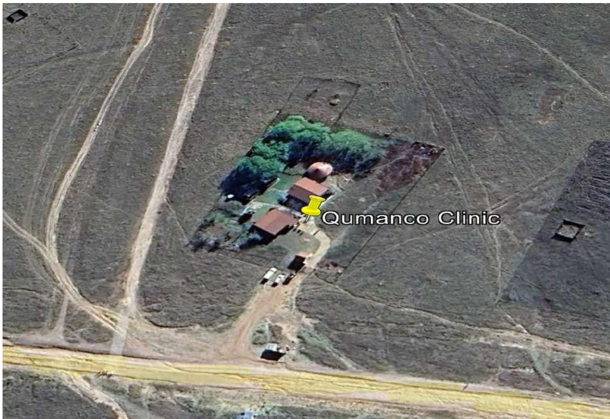
QUMANCO CLINIC AERIAL VIEW (SOURCE GOOGLE EARTH)
