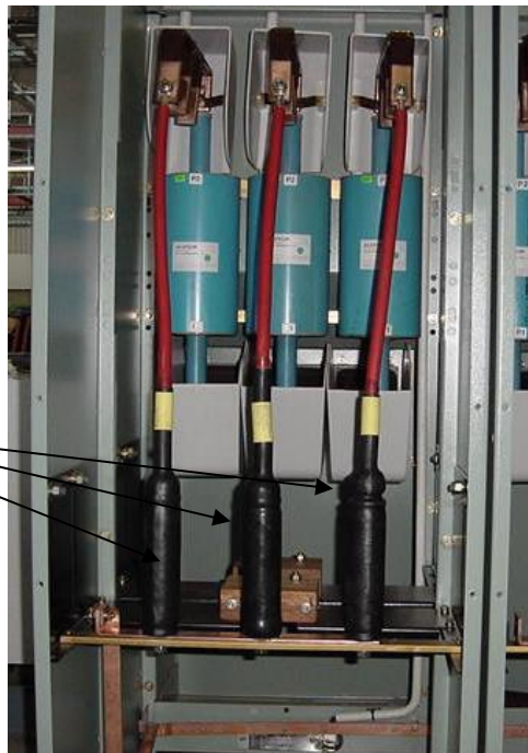
Figure A.3: 800 A feeder panel with surge arresters fitted
