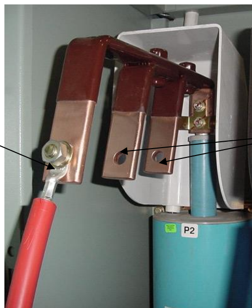
Figure A.4: Surge arrester point of attachment
