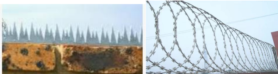
Figure 2: Image of galvanised shark-teeth spikes on top of brick wall (left); and flat wrap razor wire (right).
