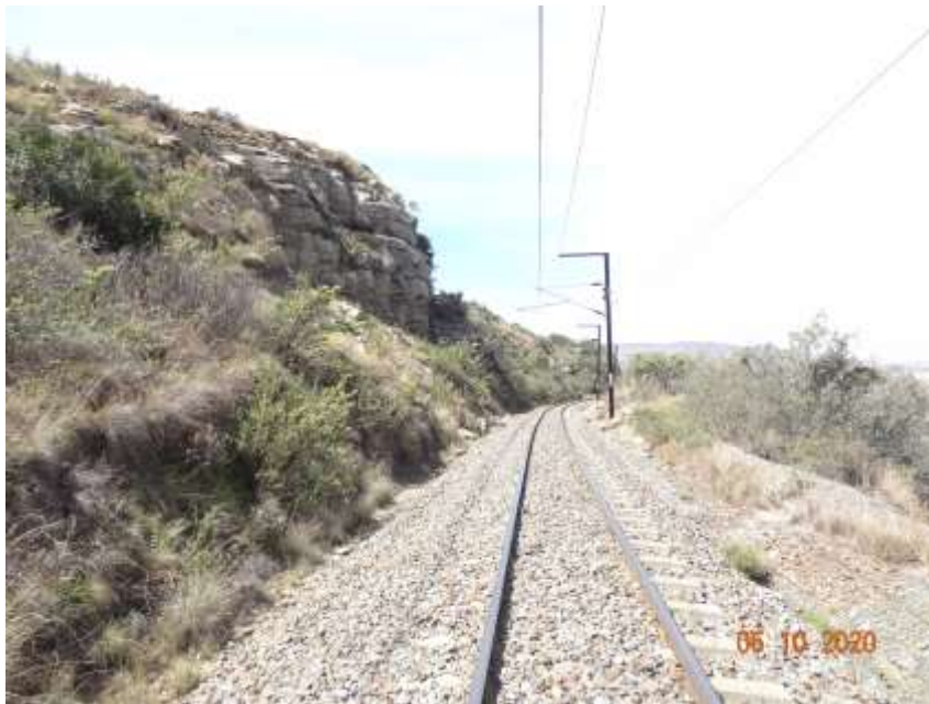
Figure 1-1: Site 1 - km 36/06, near Sterkstroom, Eastern Cape.
