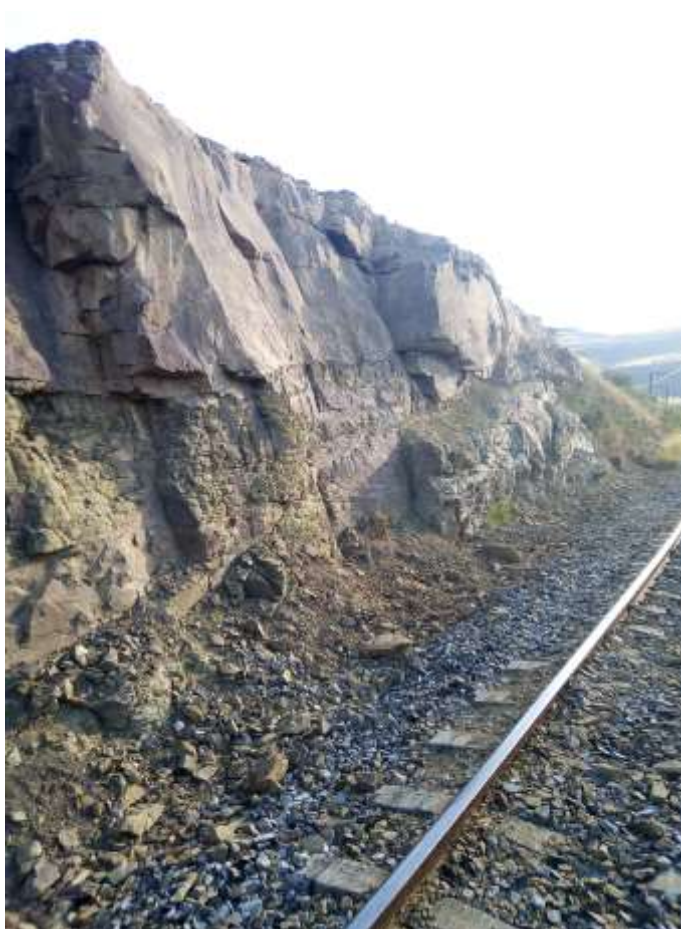
Figure 1-2: Site 2 - km 38/06, near Sterkstroom, Eastern Cape.
