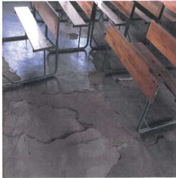
Ground floor slab shows cracks
