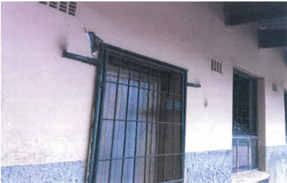
External Load Bearing wall
