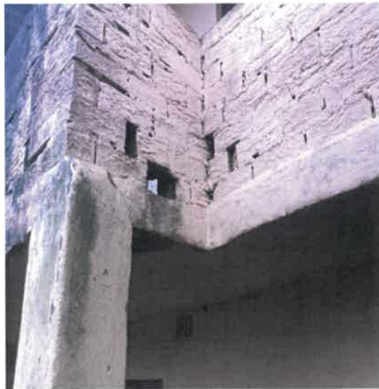
Vertical Cracks on the beams
