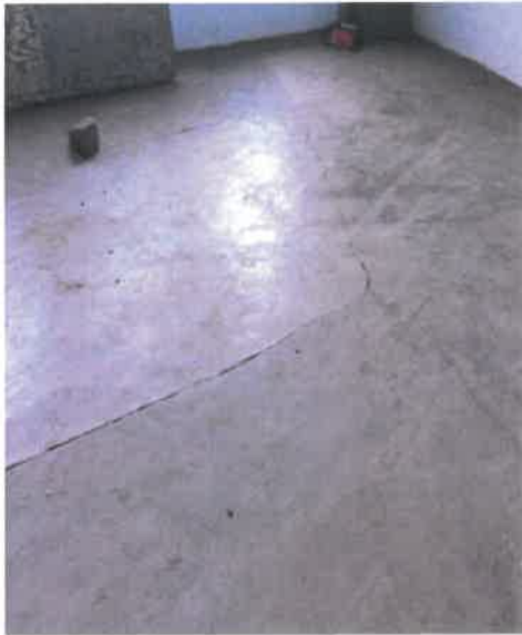
Ground floor slab shows cracks
