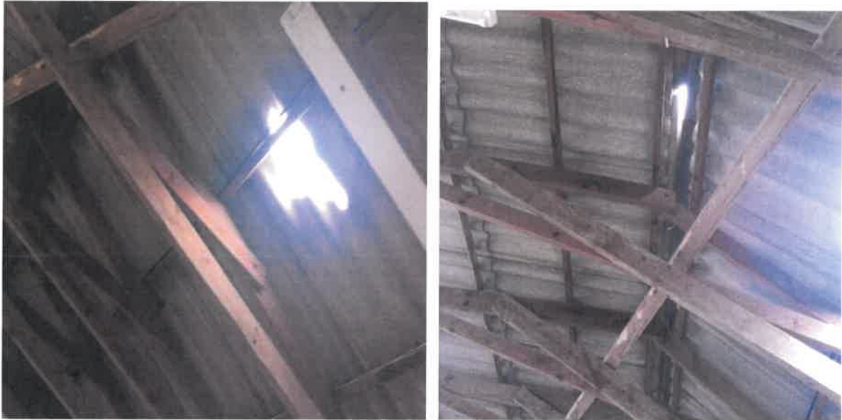
Roof Sheeting and purlin blown off and trusses damaged
