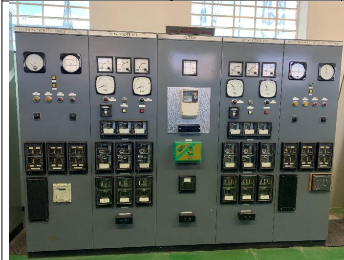
Combined Transformer No.1 and 2' tap changer and 22kV breaker control panels with indication and relays.
