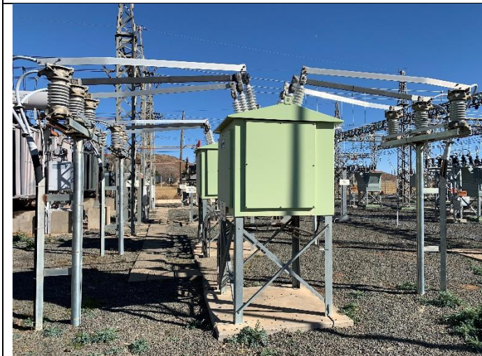
Two 22 kV "Dog Boxes" to be serviced
