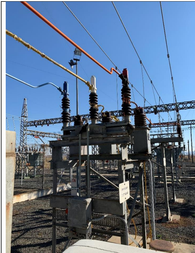
22 kV circuit breaker that needs to be serviced
