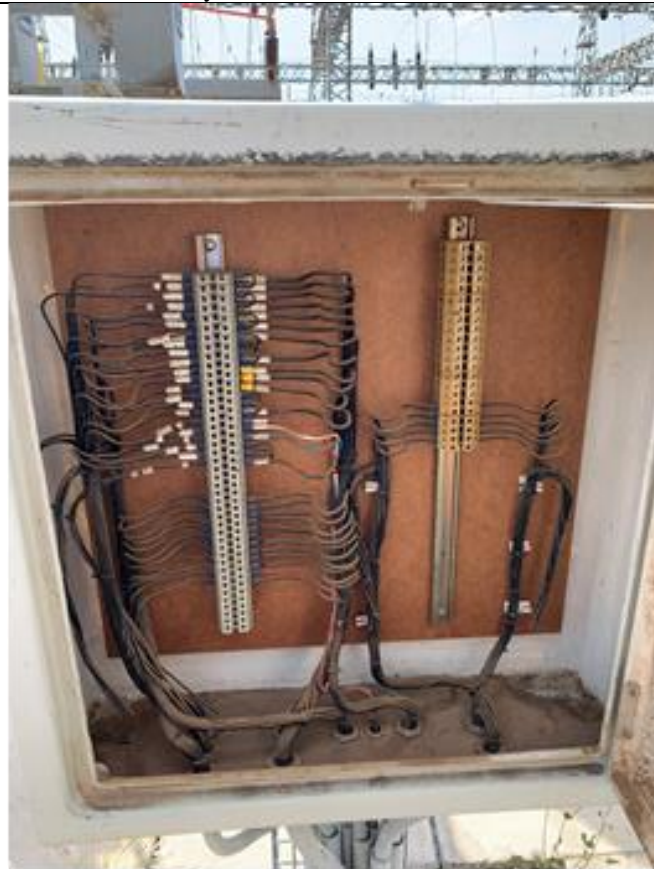
VT, CTs and circuit breaker marshalling kiosk
