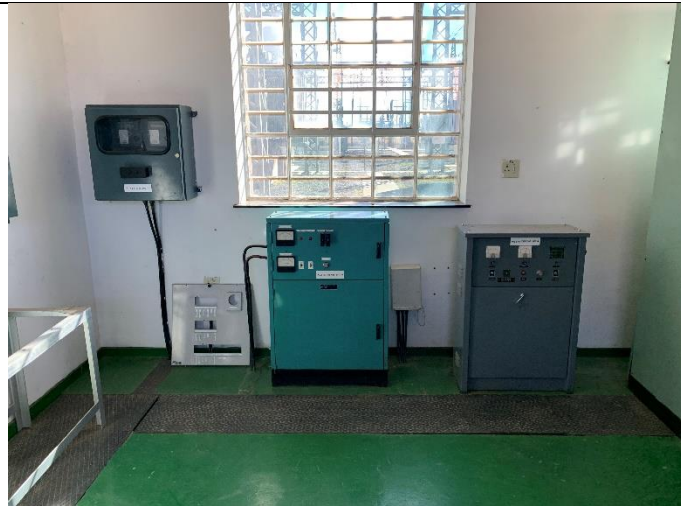
Existing BTUs that might have to be moved to make space for new control panel
