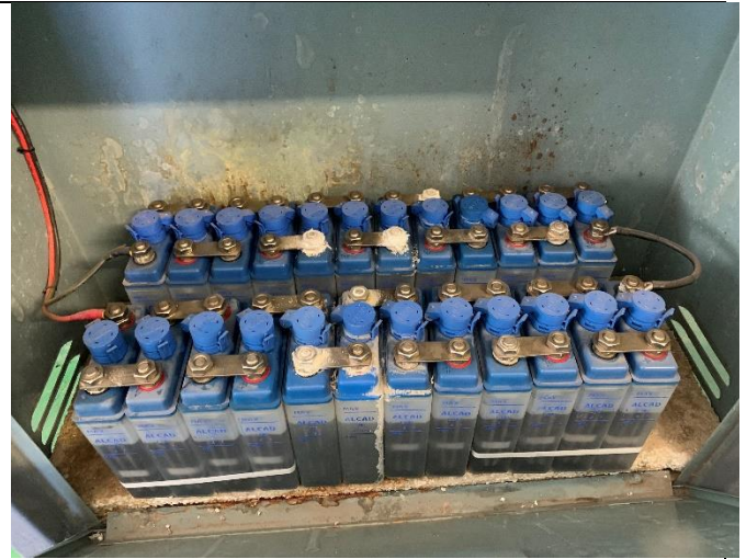
Batteries of BTU No.2 to be replaced.
