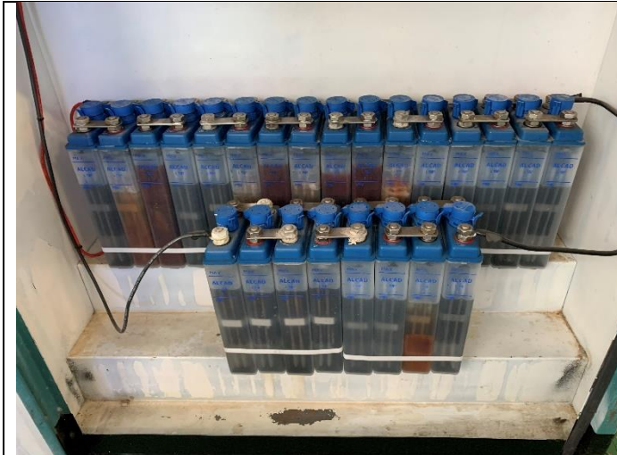
Batteries of BTU No.1 to be replaced.
