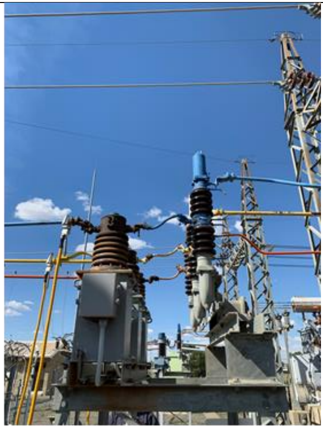
22 kV CTs and circuit breaker
