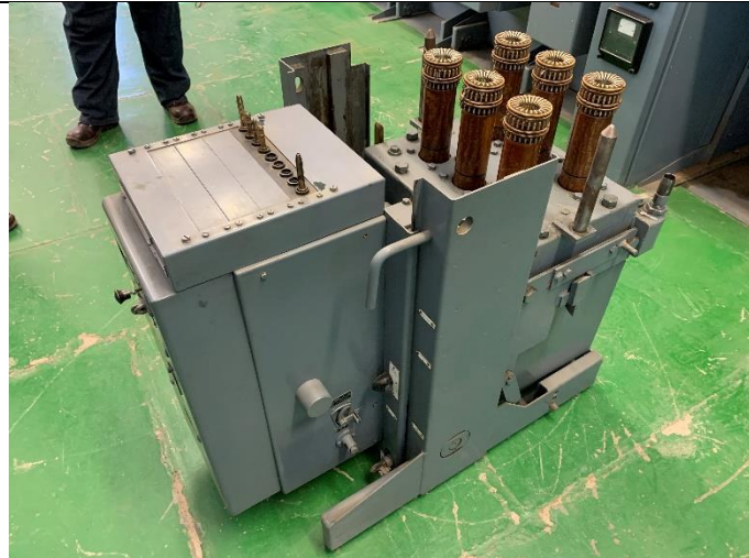
6.6 kV incomer breaker removed
