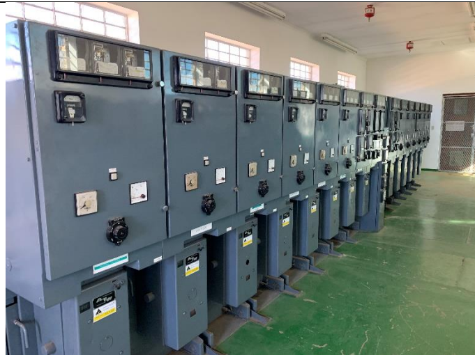
6.6 kV Switchgear Panels to be serviced
