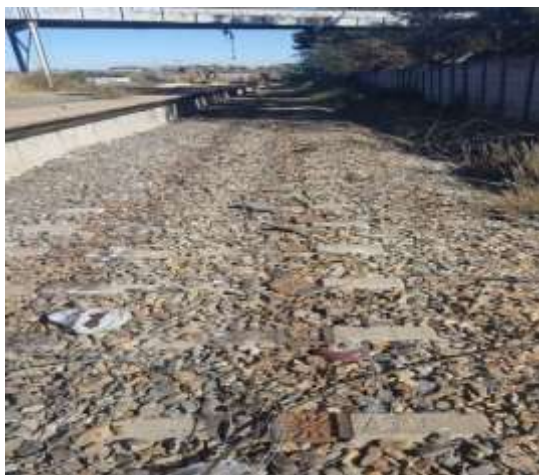
Fig 2.3: Vandalised and stolen rails
