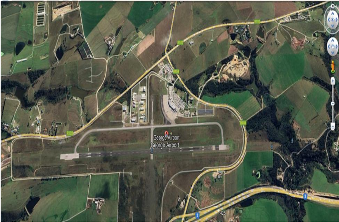
Figure C4.1: GRJ Aerial View Image
