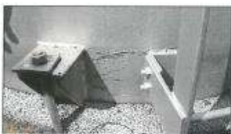
Coating failure with subsequent minor corrosion noted on tank shell.
