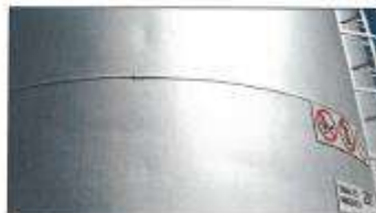
Coating failure with subsequent minor corrosion noted on tank shell.
