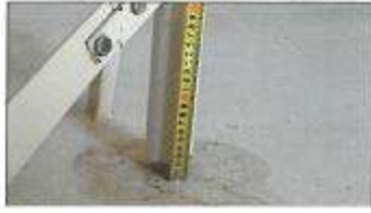
Inadequate spacing of water draw-off pipe to tank bottom.
