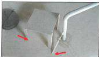
Supports welded directly to tank floor.
