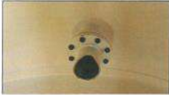
Inadequate spacing of water draw-off pipe to tank bottom.
