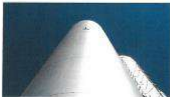
Coating failure with subsequent minor corrosion noted on tank shell.
