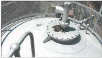
Roof plates coated with non-slip
