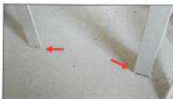
Supports welded directly to tank floor.
