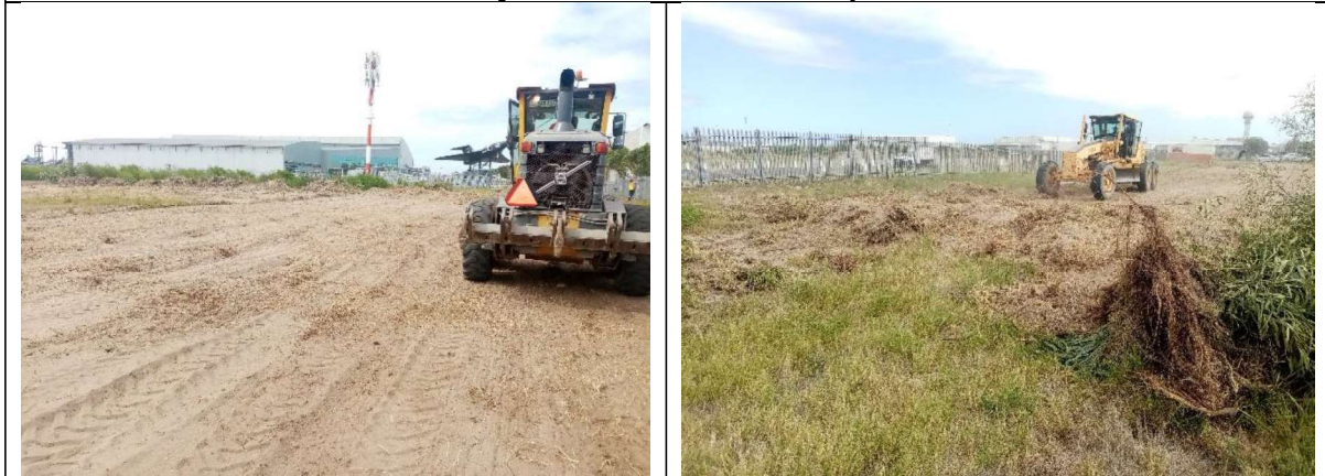
Photos showing site clearing underway
