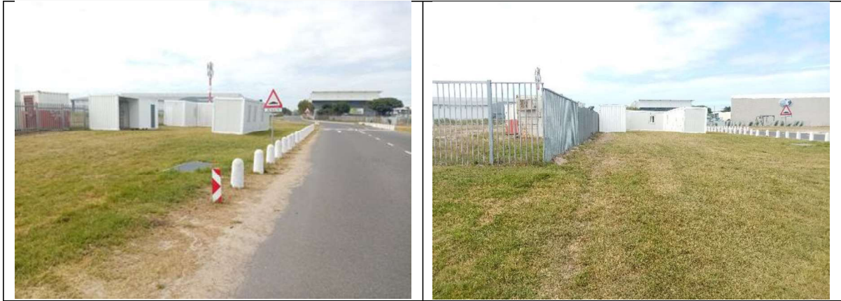
Site office being established out the site fence and adjacent to road
