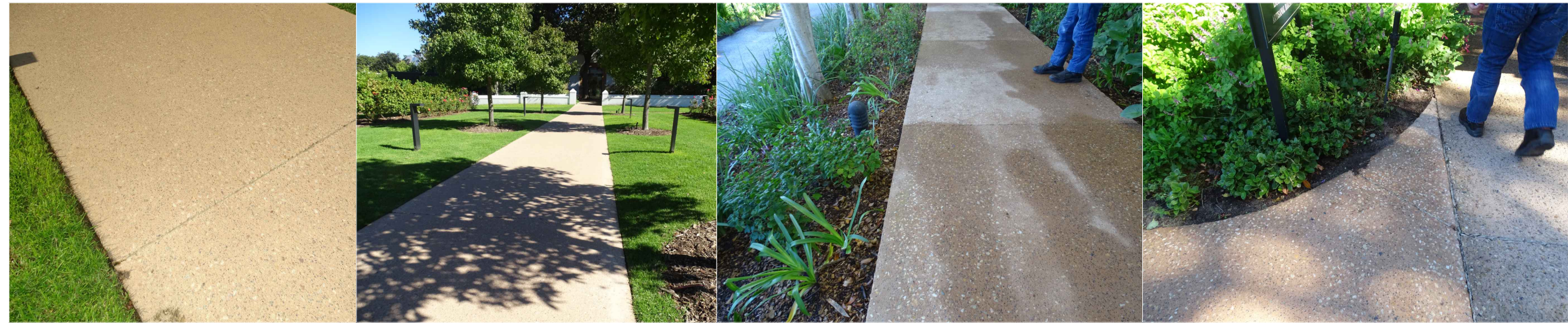
Exposed aggregate pathway Exposed aggregate pathway Exposed aggregate pathway Exposed aggregate pathway
