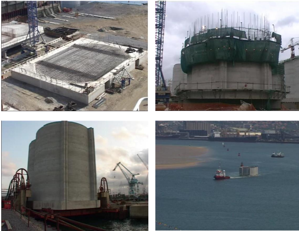
Figure 7: Caisson Construction
