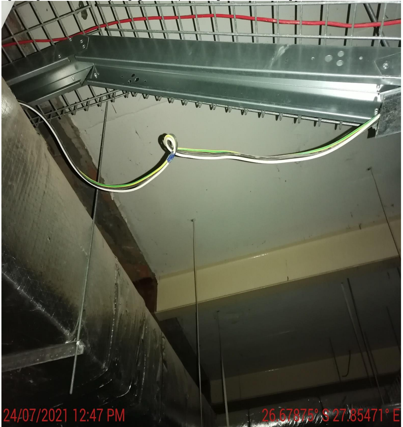
Fig 4 - Single core cables loosely hanging from the open trunking – Office 7 & 8 ceiling Void.
