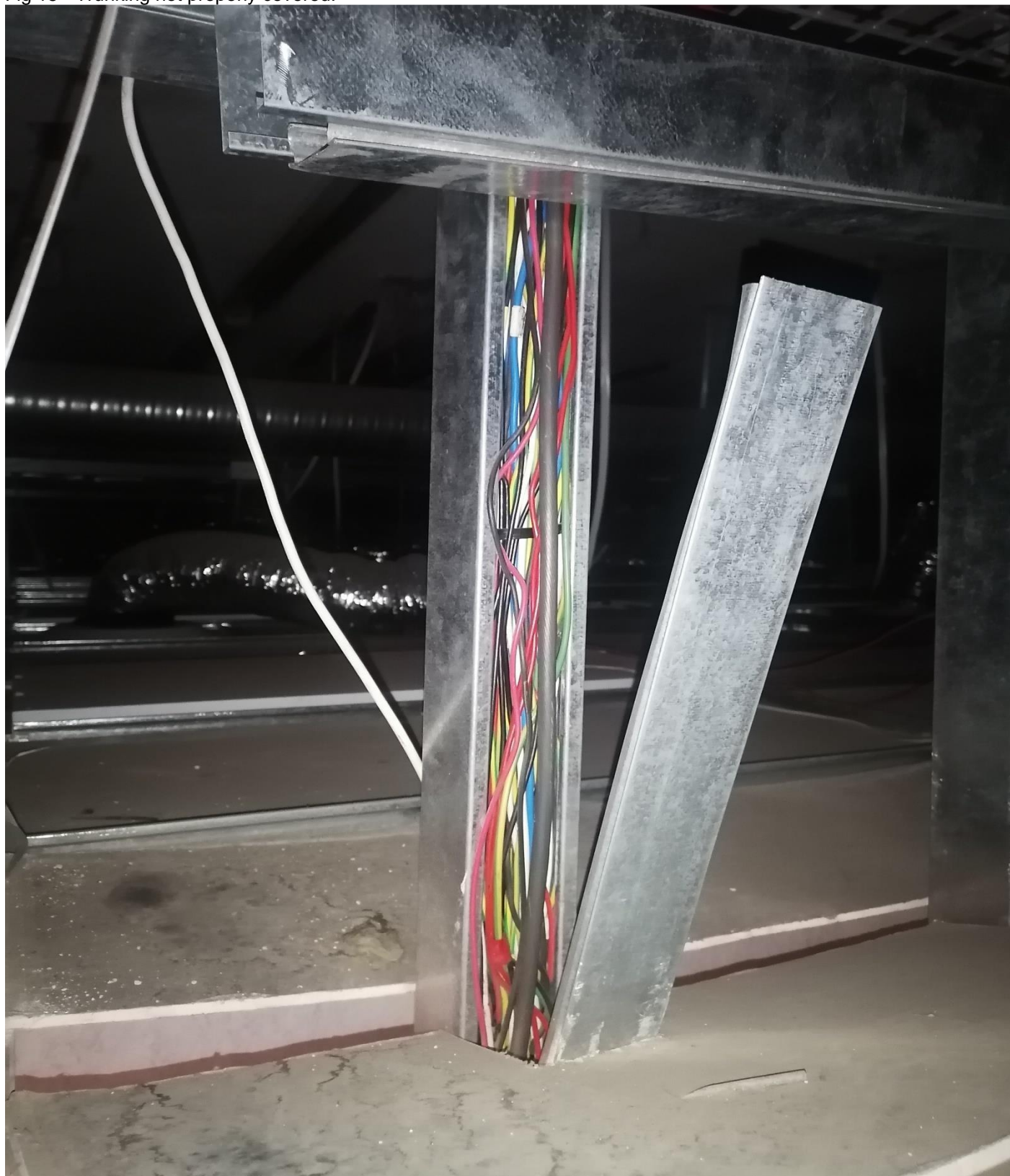
Fig 15 - Trunking not properly covered.
