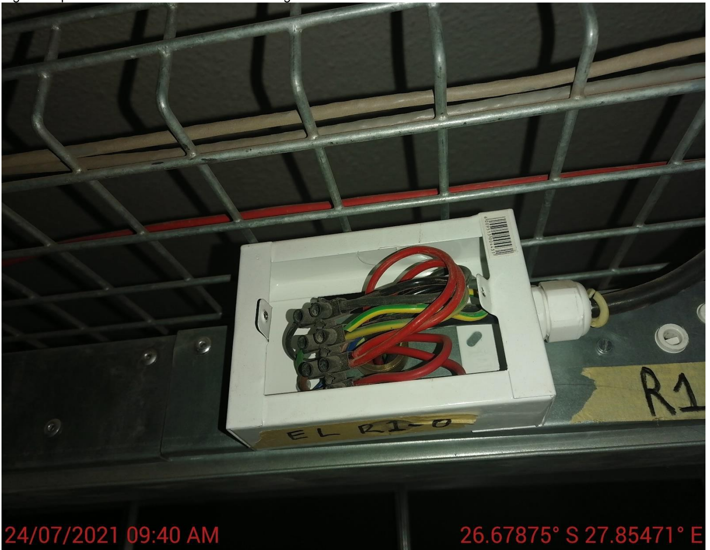
Fig 23 - Open Junction box – Tea Kitchen ceiling Void
