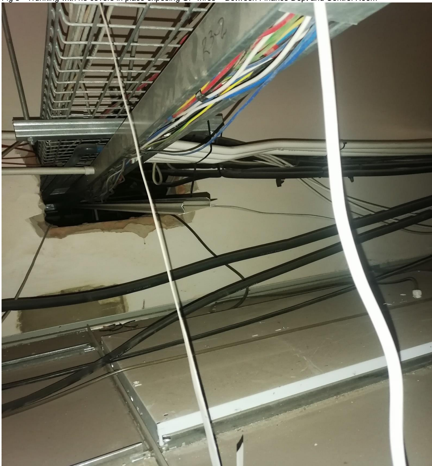
Fig 8 - Trunking with no covers in place exposing GP wires – Between Finance Dept and Control Room
