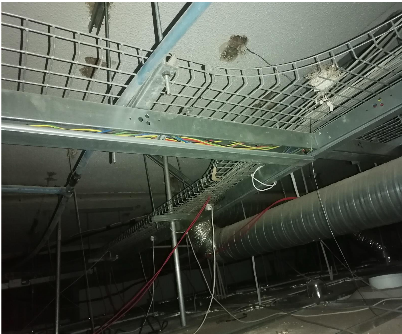
Fig 9 - Cable trunking with open covers - Entrance passage
