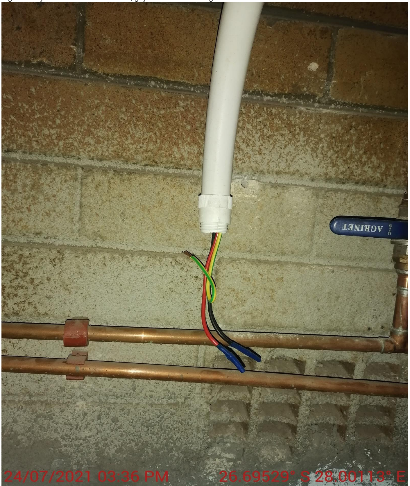
Fig 16 - Geyser cables not connected, geyser isolator missing – Female Toilets
