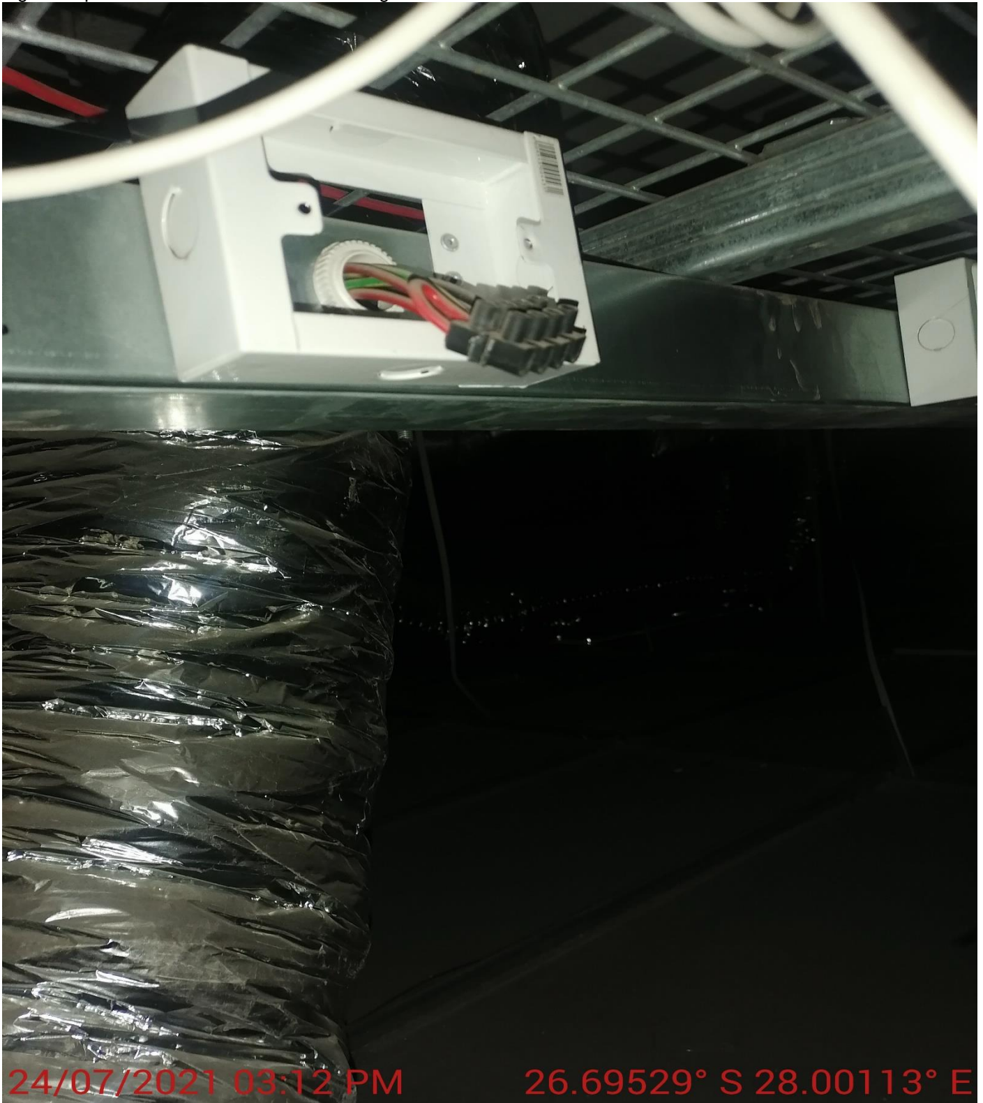
Fig 19 - Open Junction Boxes inside the ceiling void
