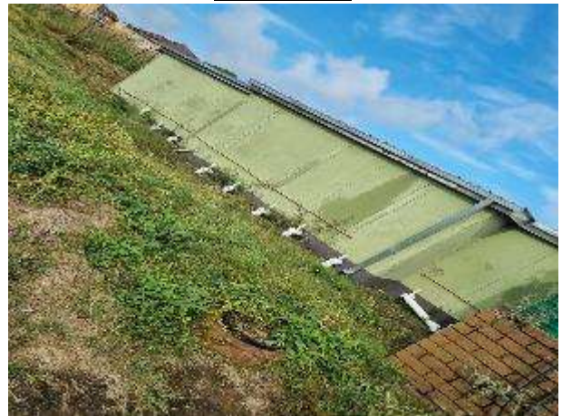
BACK VIEW OF ABLUTION BLOCK
