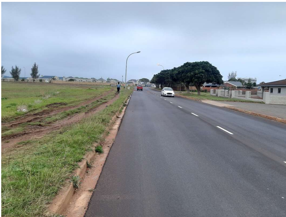
Figure 5: The site is bordered by Nautilus Street to the east. This road belongs to Kouga Local Municipality.
