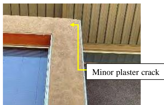
Figure 5: Showing plaster crack on the existing external wall
