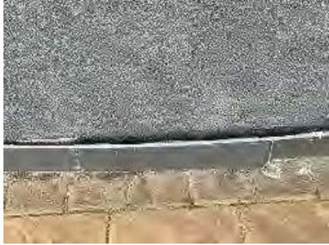
Figure 30: Showing delamination of the tiled skirting on the existing wall
