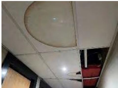
Figure 34: Showing water damage to existing ceiling boards
