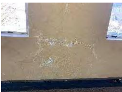
Figure 27: Showing water damage to existing internal office walls
