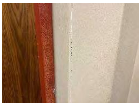
Figure 23: Showing minor plaster crack on the existing wall
