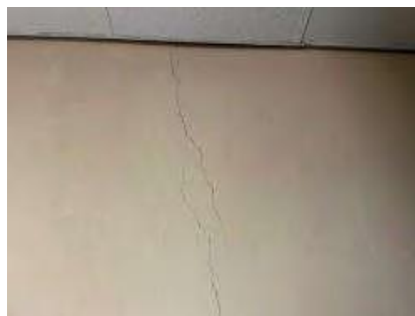
Figure 22: Showing minor plaster crack on the existing wall
