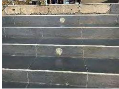
Figure 31: Showing damage to the exterior tiling
