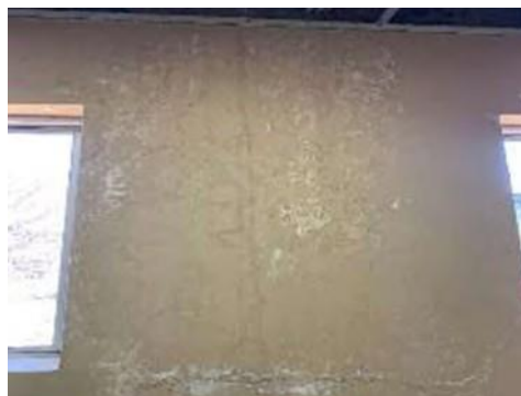
Figure 26: Showing water damage to the existing internal office wall
