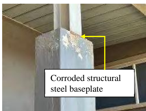
Figure 16: Showing corroded structural steel baseplate
