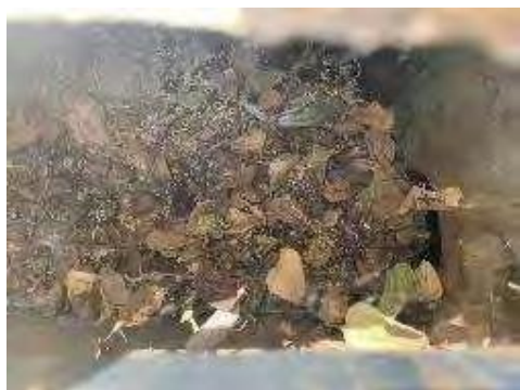
Figure 12: Showing stormwater manhole blocked with silt and debris
