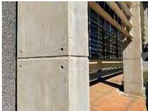
Figure 32: Showing minor spalling on the finish of the existing
