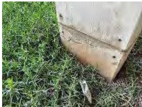
Figure 33: Showing minor spalling on the finish of the existing
