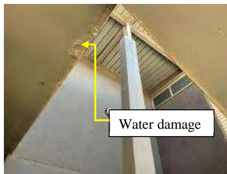
Figure 15: Showing water damage to the fire escape staircase
