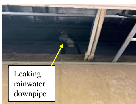
Figure 28: Showing leaking/damaged rainwater downpipe
