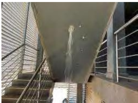
Figure 14: Showing water damage to the existing fire escape staircase
