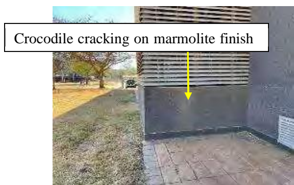
Figure 4: Showing minor cracking of the existing marmolite finish
