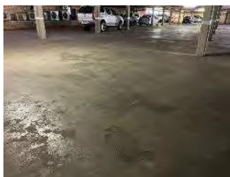
Figure 19: Showing damage to existing concrete surface bed slab at basement level
