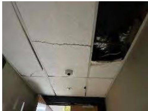
Figure 35: Showing cracked/damaged ceiling boards
