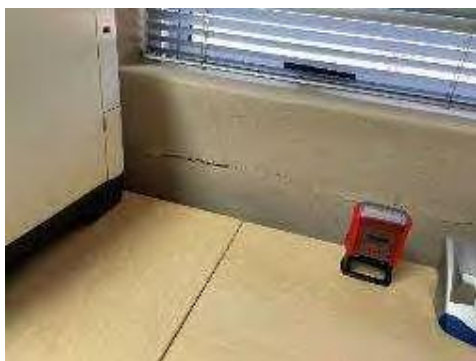
Figure 25: Showing minor horizontal plaster crack on the existing wall
