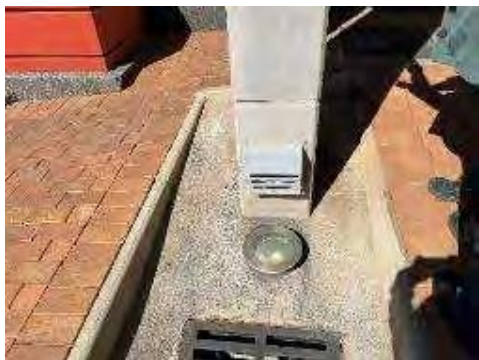
Figure 10: Showing rainwater downpipe grid inlets
