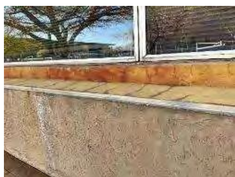
Figure 6: Showing plaster cracks on the existing external wall.
