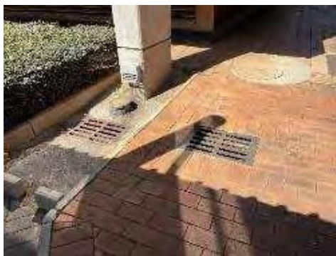
Figure 13: Showing existing stormwater grid inlets
