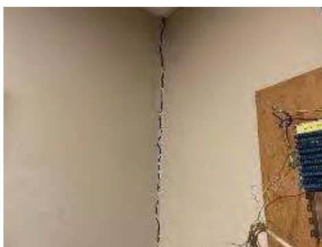
Figure 24: Showing moderate plaster crack on the existing wall
