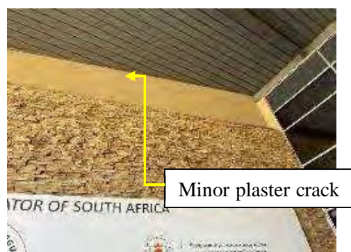
Figure 7: Showing plaster crack on the existing external wall.
