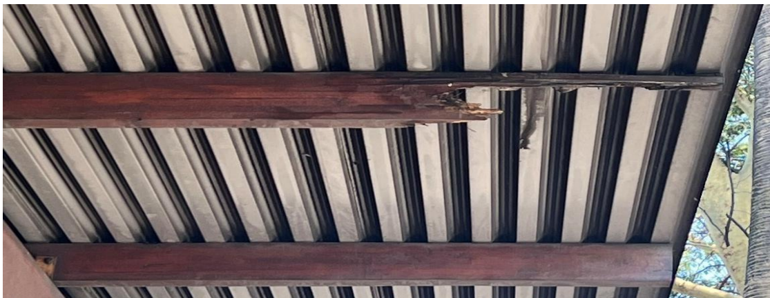
Figure 2: Damaged Timber Batten
