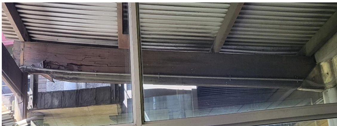
Figure 1: Damaged Timber Rafter
