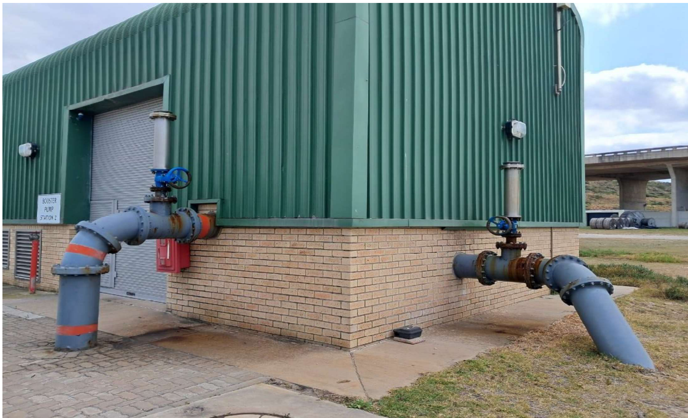
Figure 5: One of the four booster stations with exposed inlet and outlet Jet pipes
