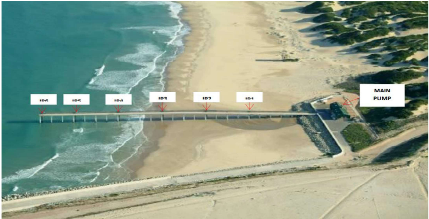
Figure 4: Aerial view of Sand Bypass Jetty, showing the full length of pipeline including all Jet pumps (JP1 to JP6)
