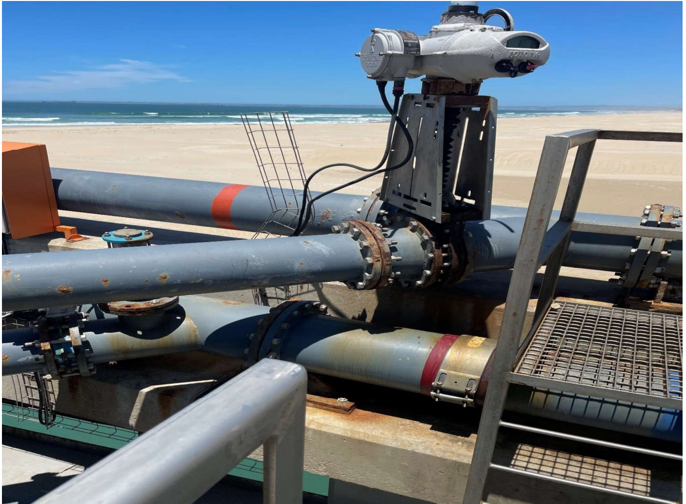
Figure 9: Pipeline with gate valve and actuator
