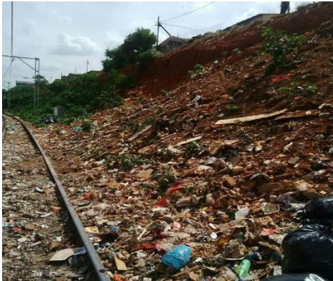
The sleepers not visible and covered by the garbage at Limindlela
