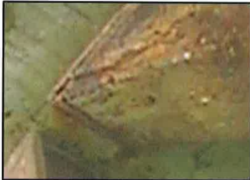
A - Line Crack line Spine beam.
