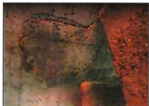
Delamination/Honeycombing B3 - B1
