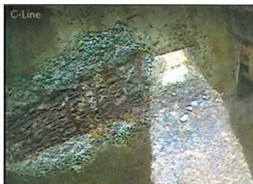
C - Line slab and pile delamination. Group 23
