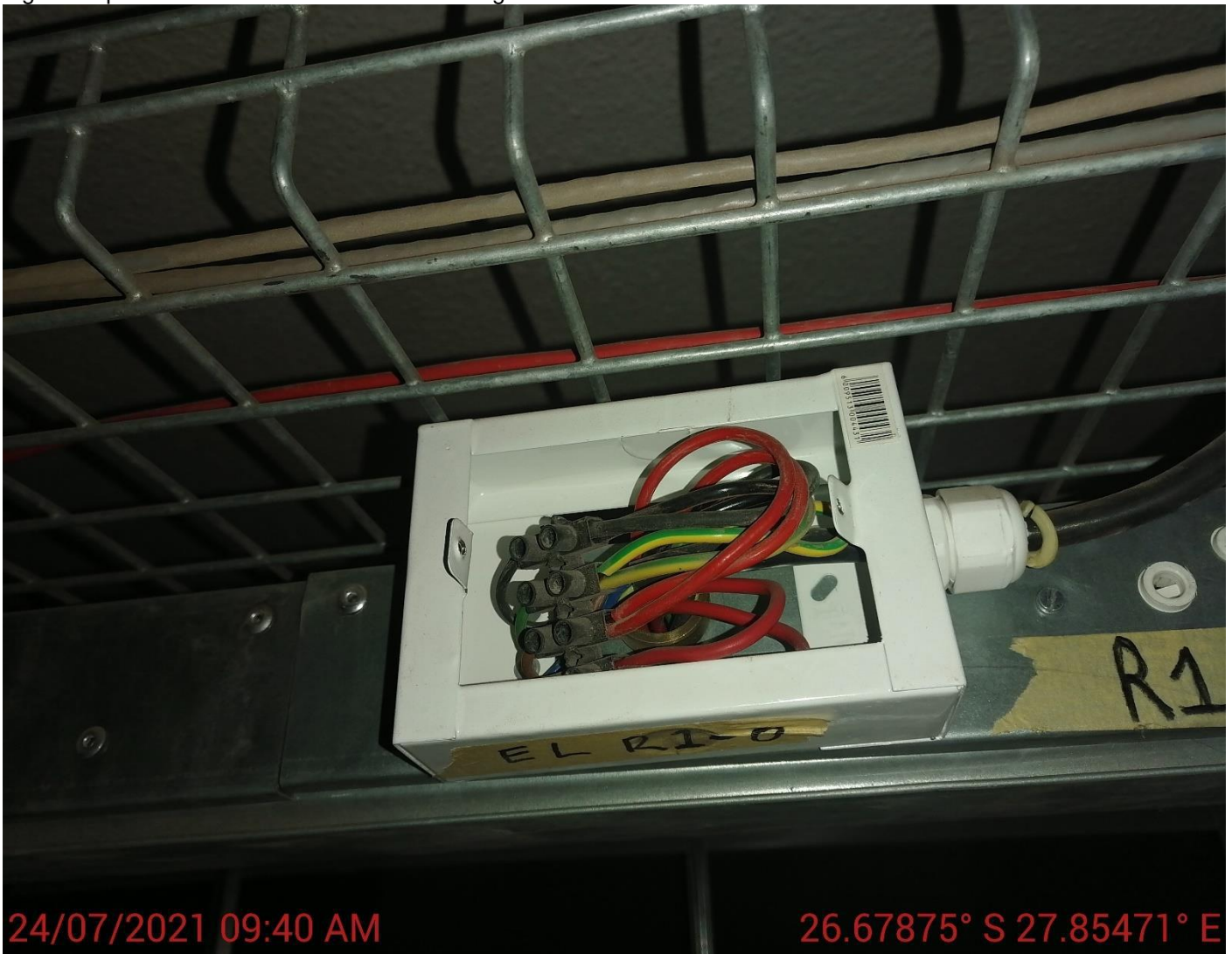
Fig 23 - Open Junction box – Tea Kitchen ceiling Void
