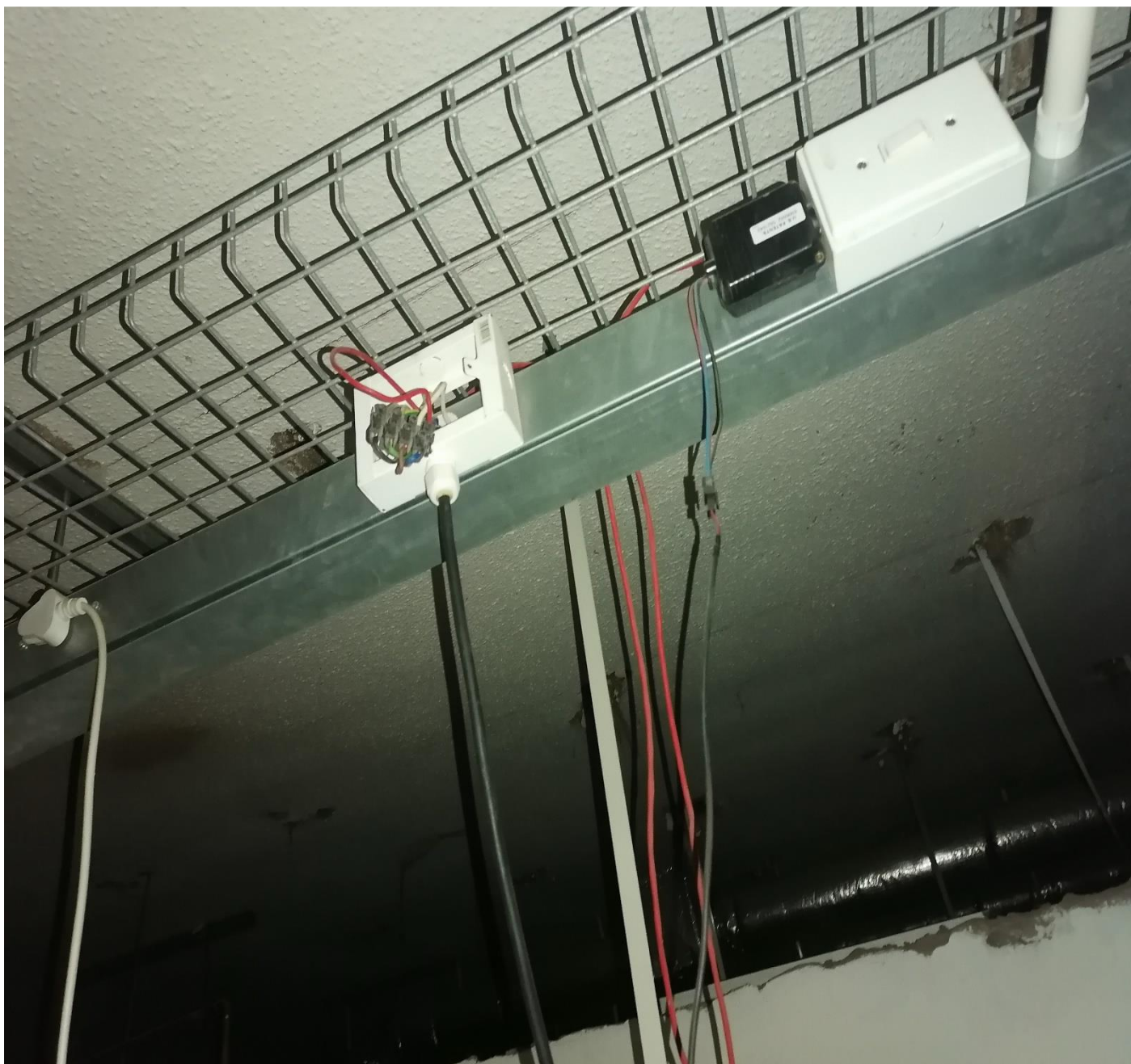
Fig 7 - Open junction boxes exposing connections – Open Plan next to Financial Admin Office
