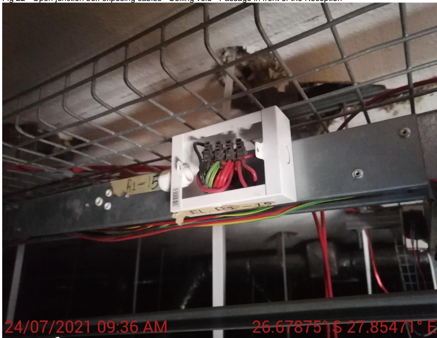
Fig 22 - Open junction box exposing cables– Ceiling void - Passage in front of the Reception
