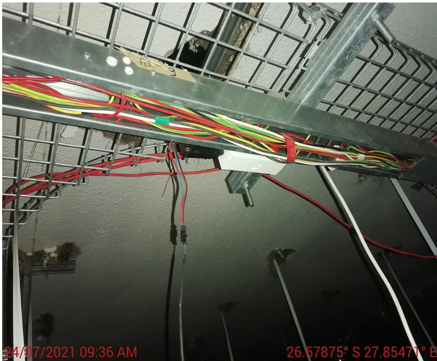
Fig 1 - Open trucking covers inside the ceiling exposing GP wires – Reception Ceiling Void
