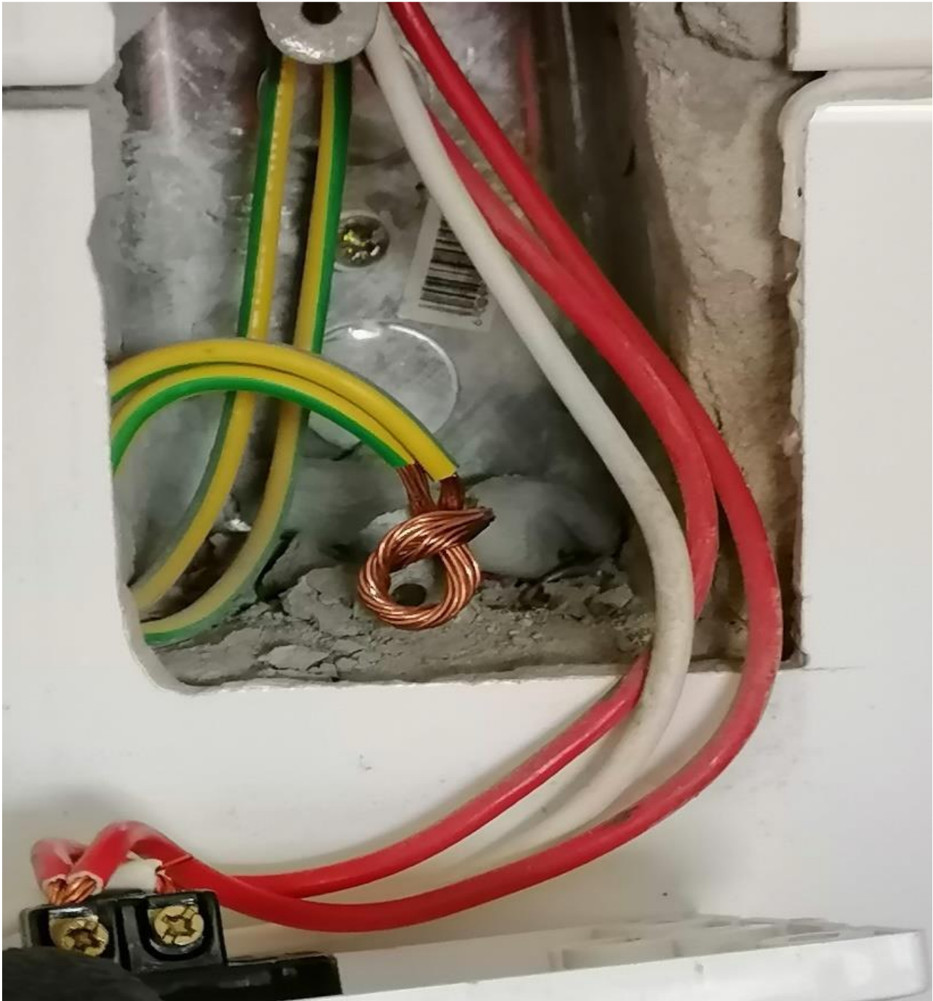
Fig 27 – Improper earth terminations on switch boxes. Tea Kitchen Switch
