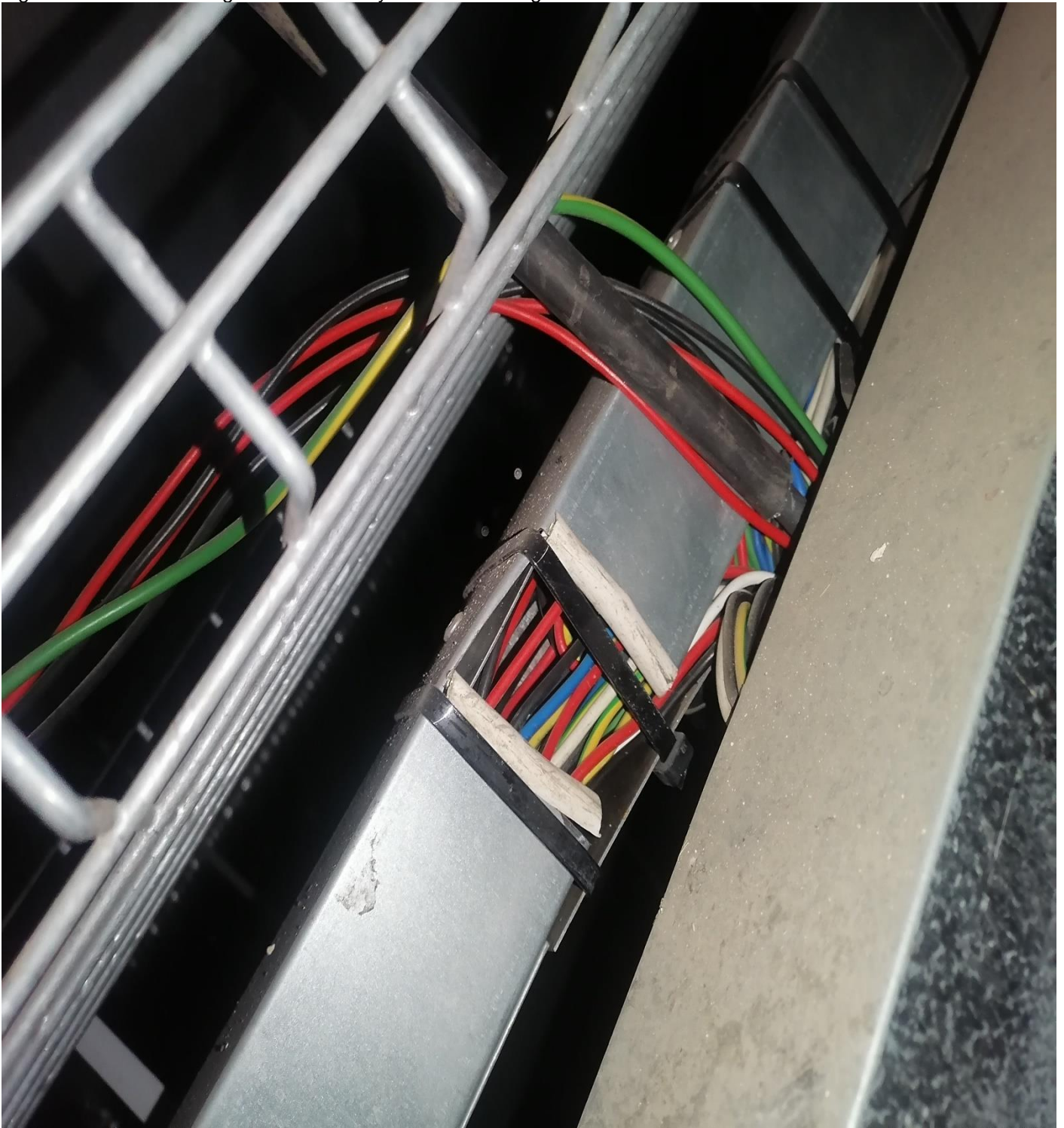
Fig 20 - GP Wires running on the cable tray inside the ceiling.
