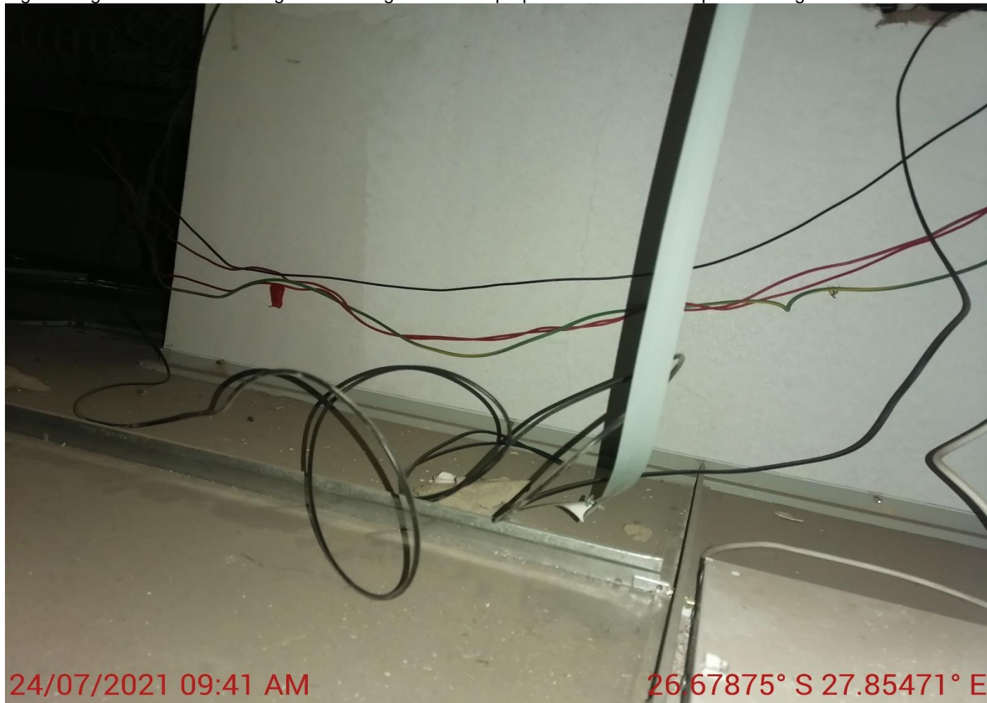
Fig 2 - Single core cables running in the ceiling without the proper enclosure – Reception Ceiling Void
