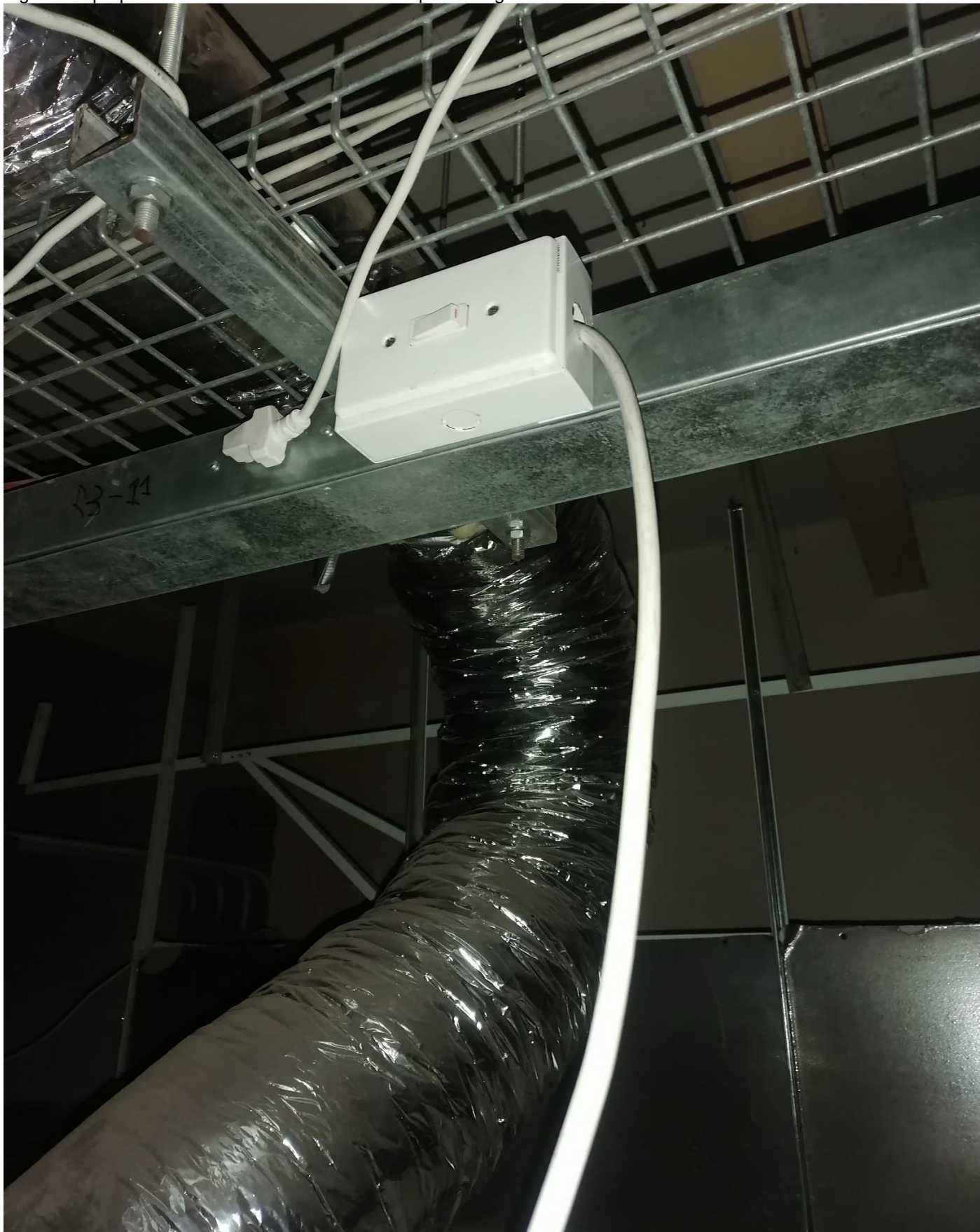
Fig 26 - Improper Cable termination – without compression glands
