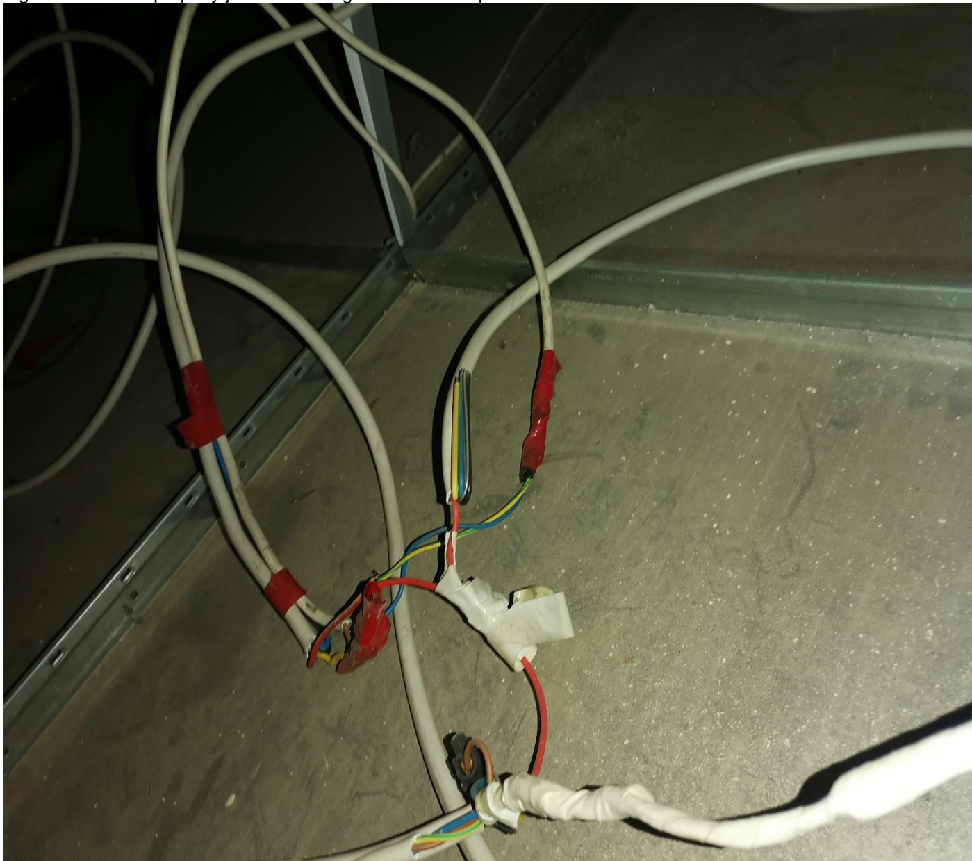
Fig 10 - Cables improperly joined – Ceiling Void above Supervisor's Office
