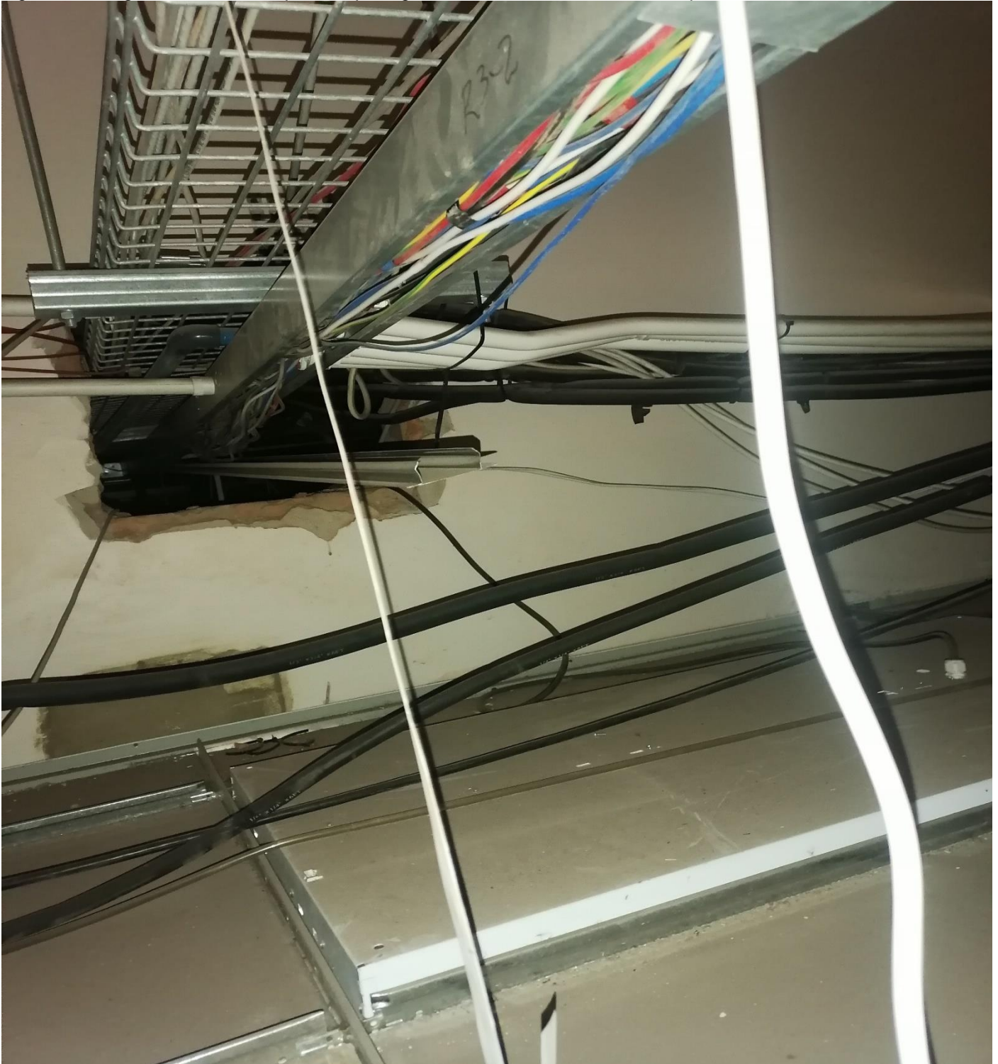
Fig 8 - Trunking with no covers in place exposing GP wires – Between Finance Dept and Control Room
