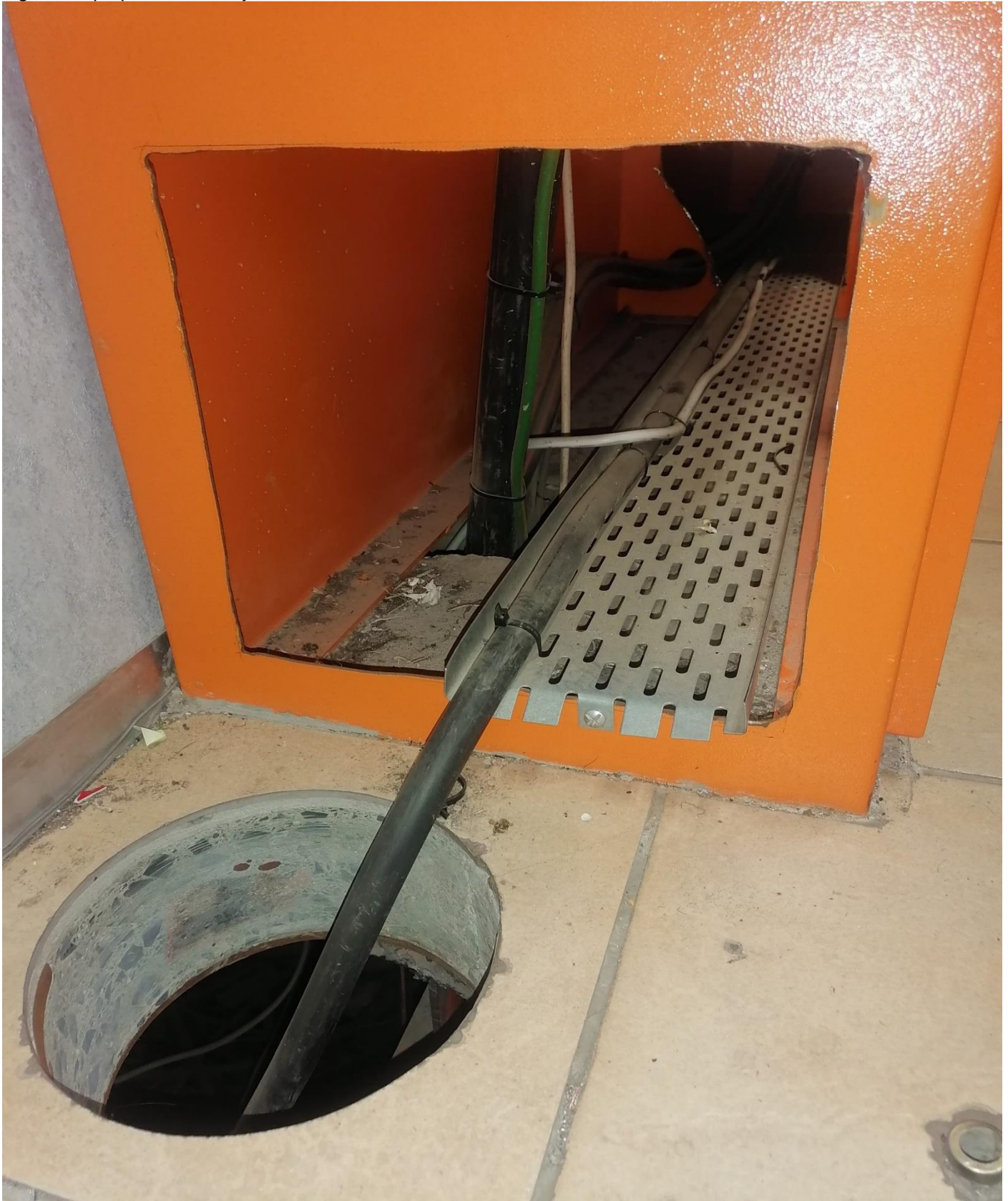
Fig 18 - Improper Cable entry into the DB – Electrical Room
