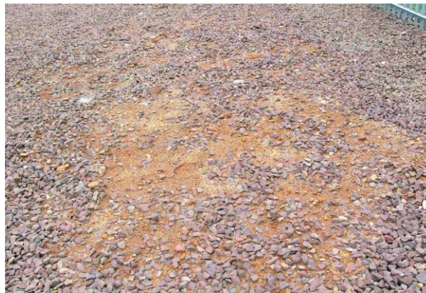
Figure 14: Exposed soil due to poor workmanship
