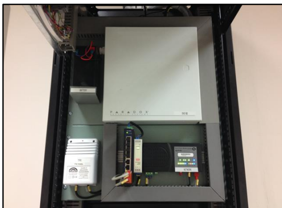
Figure 8: Example of Well Organised Security Equipment Cabinet
