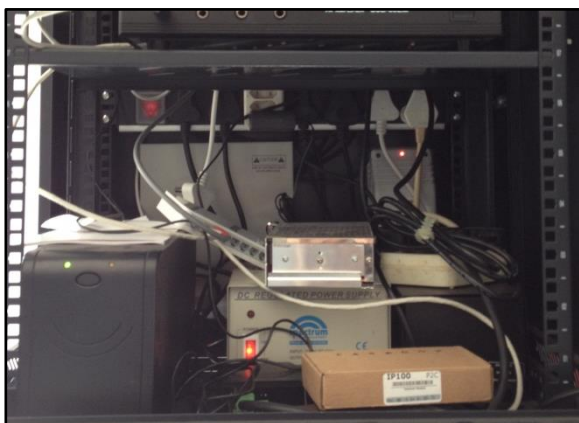
Figure 7: Example of Poorly Organised Security Equipment Cabinet
