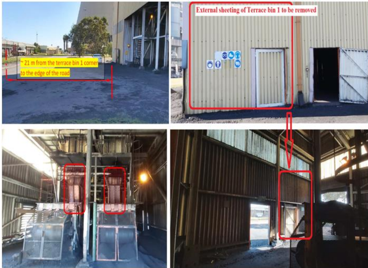
Figure 3: Modification of TB1 Housing for Cooling operations
