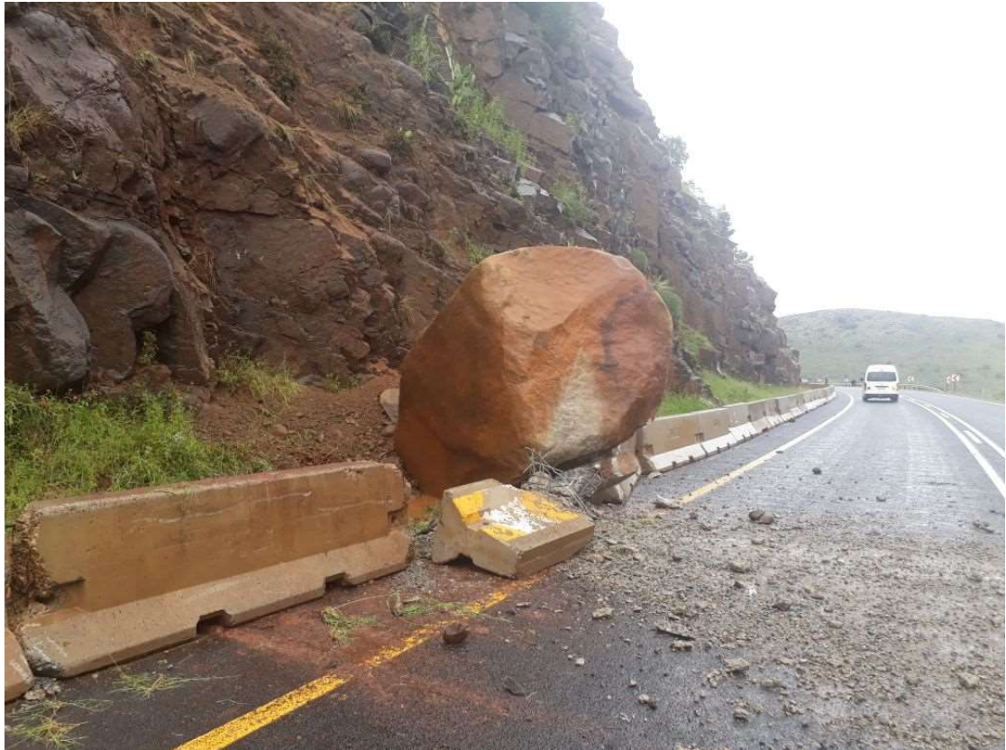
Figure C4.11-1: Dolerite corestone that dislodged and crushed a new jersey barrier on 8 March 2018
