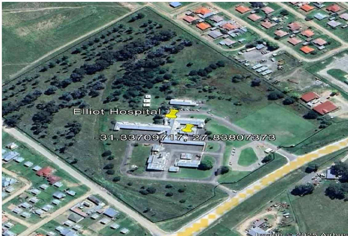
ELLIOT HOSPITAL AERIAL VIEW (SOURCE GOOGLE EARTH)
