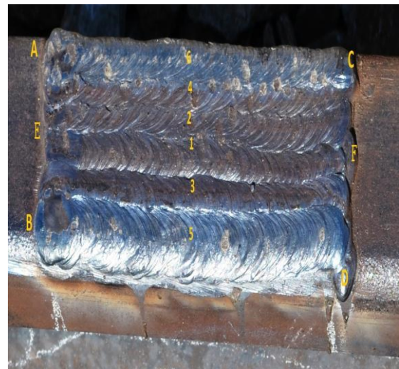
Figure 5: Skid mark repaired by open-arc welding
