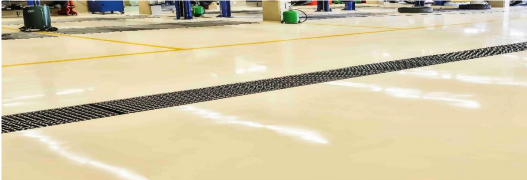
Example of epoxy floor
