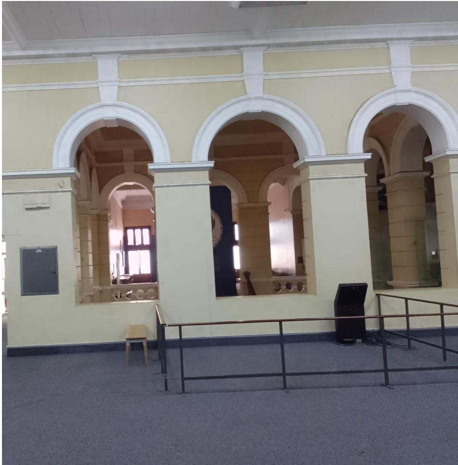
Figure 5. Install three large frameless glass panes between pillars near staircase
