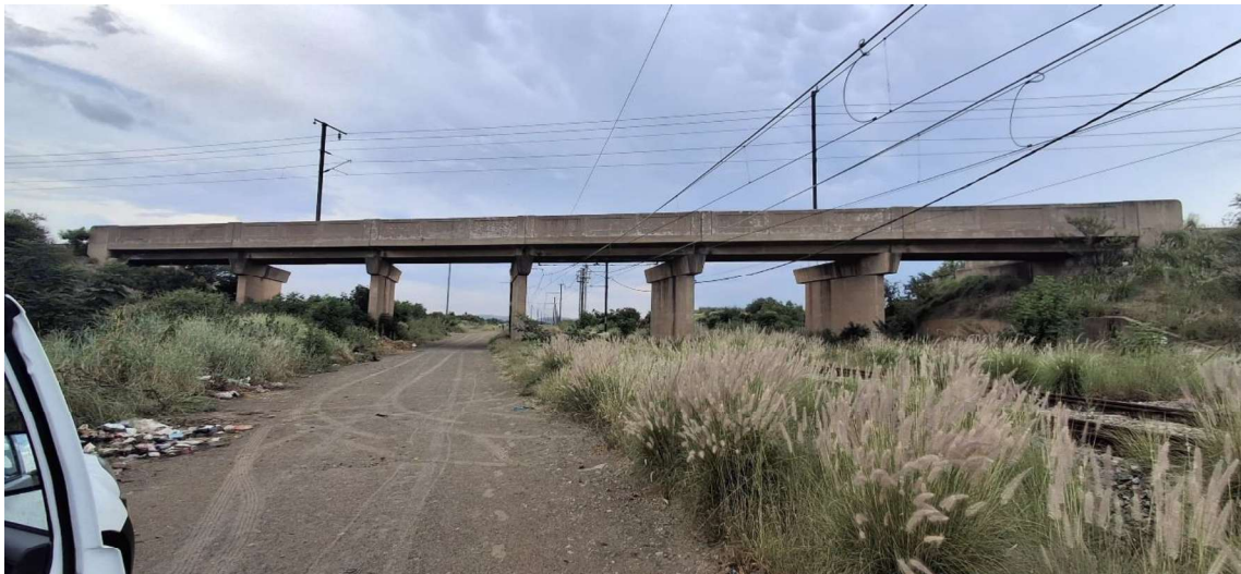
Pyramid South Concrete Bridge FRP Handrail Km 16/17 75m
