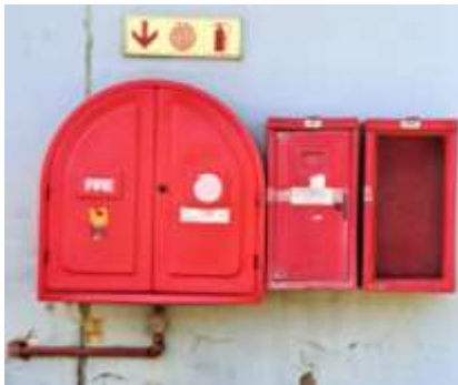
Hose reels with associated pipework and fittings (Maintenance Buildings, Fire Station, Fuel Depo)
