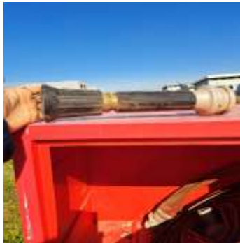
43 x Fire Hydrant Hoses (inclusive of couplings and 1 x branch per cabinet) in UV-Resistant Red plastic Fire Hydrant cabinets
