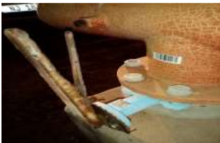
2 x Fire Hydrant butterfly valves Replacement and painting of hydrants
