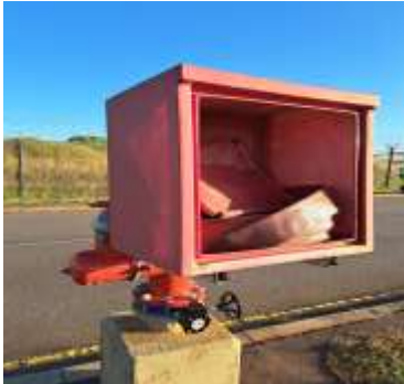
43 x Fire Hydrant Hoses (inclusive of couplings and 1 x branch per cabinet) in UV-Resistant Red plastic Fire Hydrant cabinets
