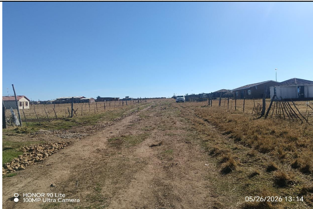
Virgin road with uncontrolled stormwater causing erosion
