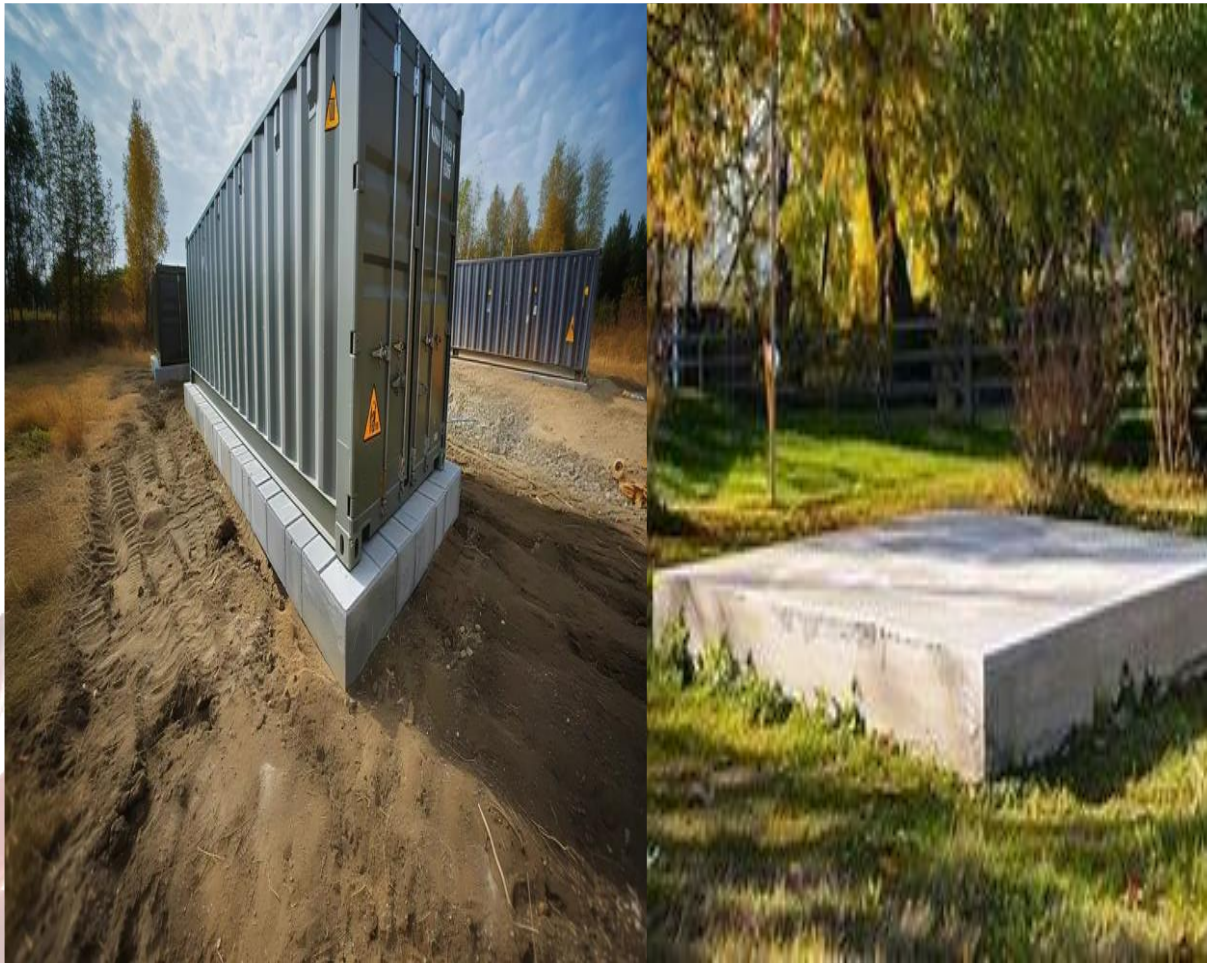
Concrete foundation for storage facility
