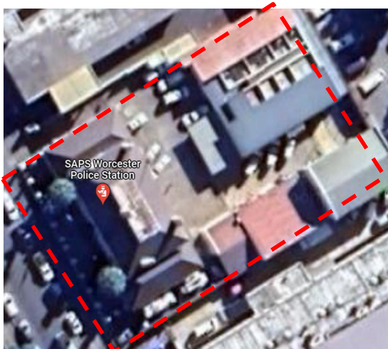
Figure 1: Aerial View of Worcester Police Station
