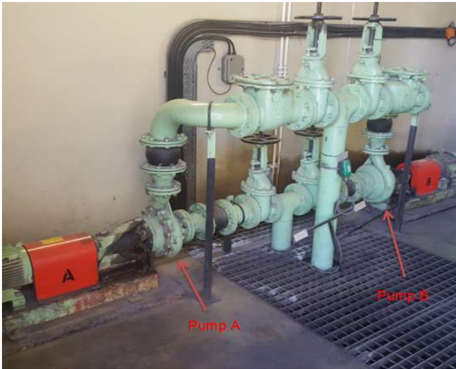
Figure 7: Cooling Water Pump Layout
