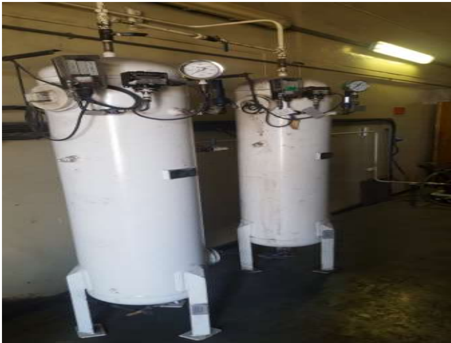
Figure 5: Existing Air Receivers
