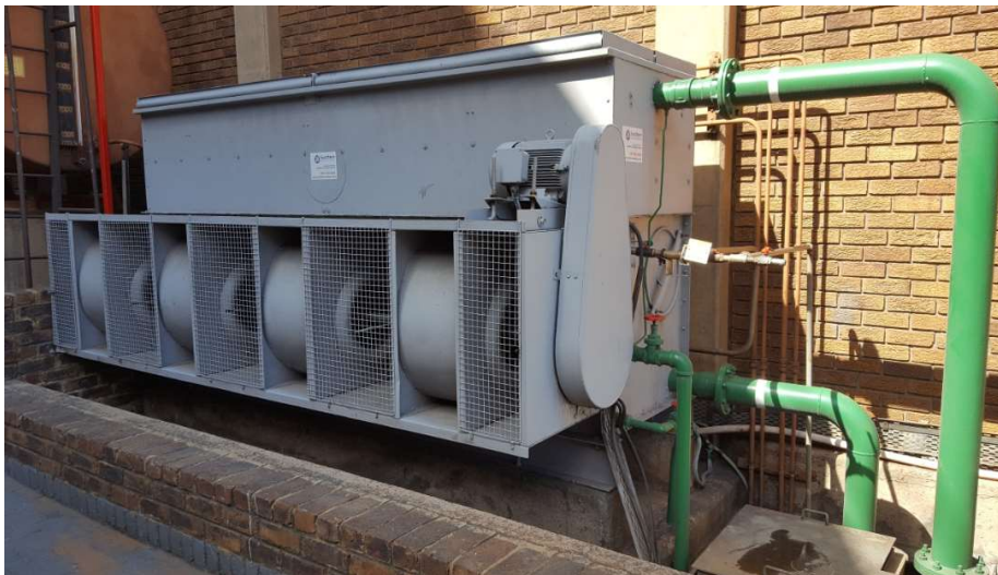
Figure 6: Cooling Tower
