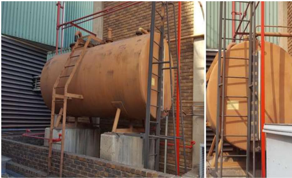
Figure 8: Diesel Storage Tank and Level Indication
