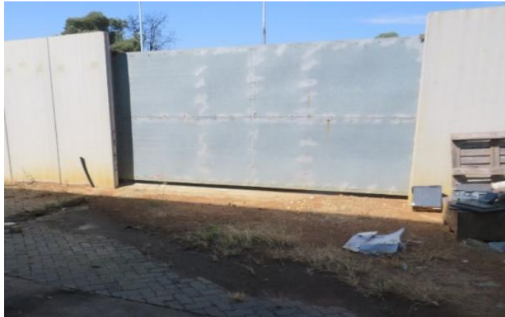
Figure 2 Alrode Vehicle Access Gate
