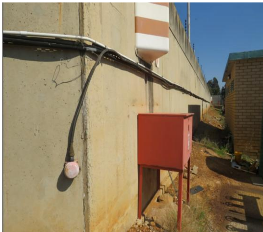
Figure 3 Fire Emergency Box (Left); Loose Electrical Cabling (Right)
