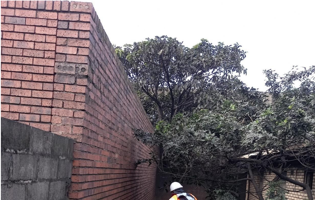
Photo of a tree growing adjacent to the Bund-wall
