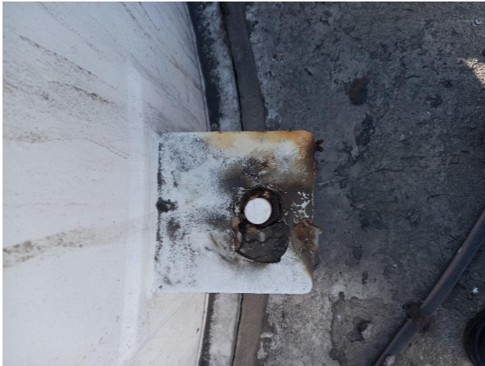
Tank Anchor Chair is severely corroded
