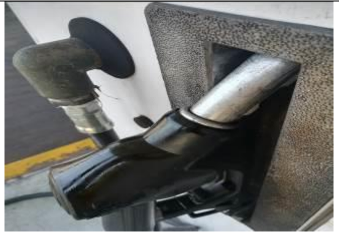
Nozzle leaking needs repairs
