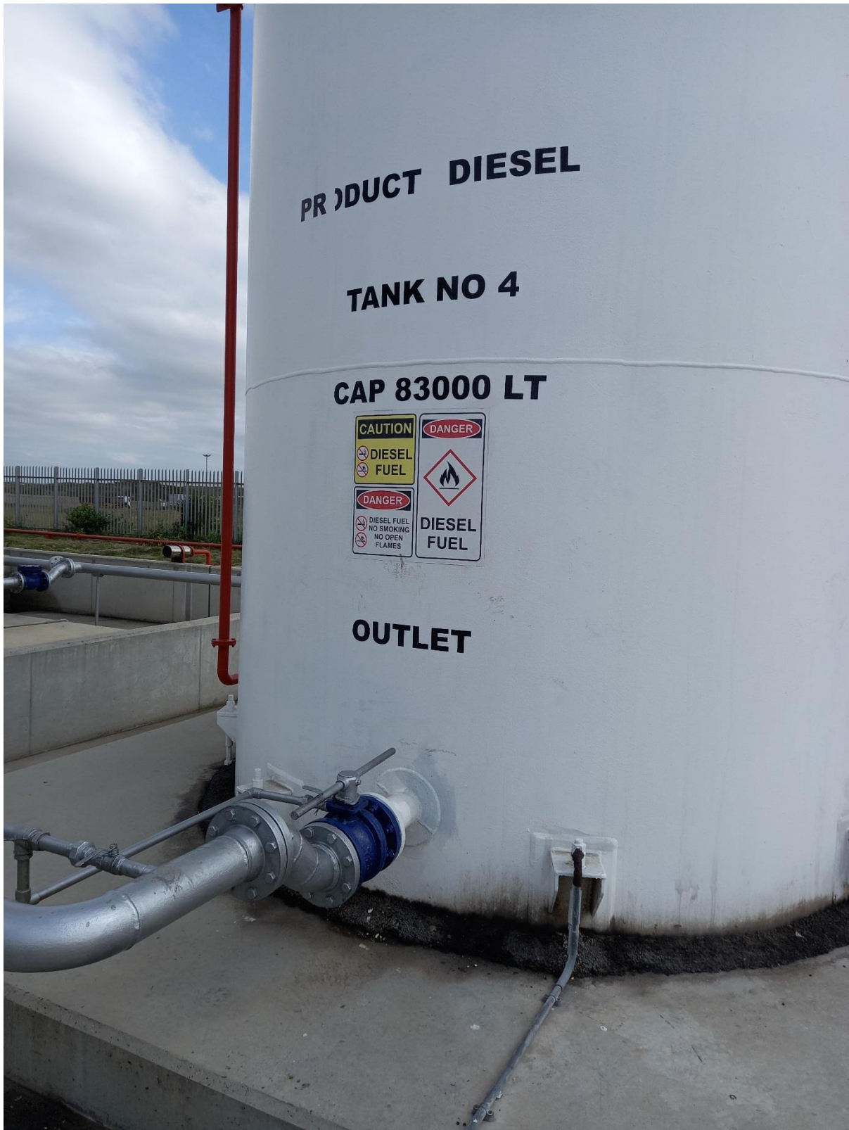
Close up photo of tanks with annular ring, earthing cables and outlet nozzle
