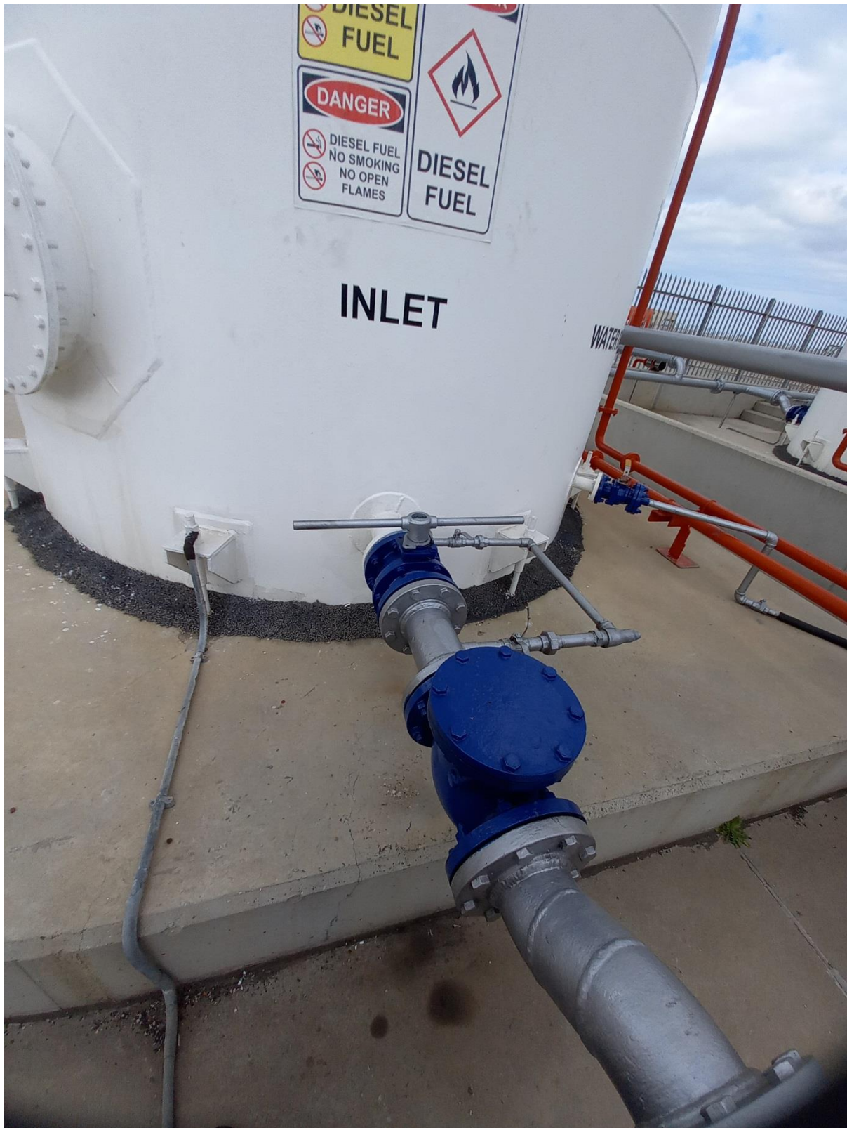
Tank Inlet nozzle
