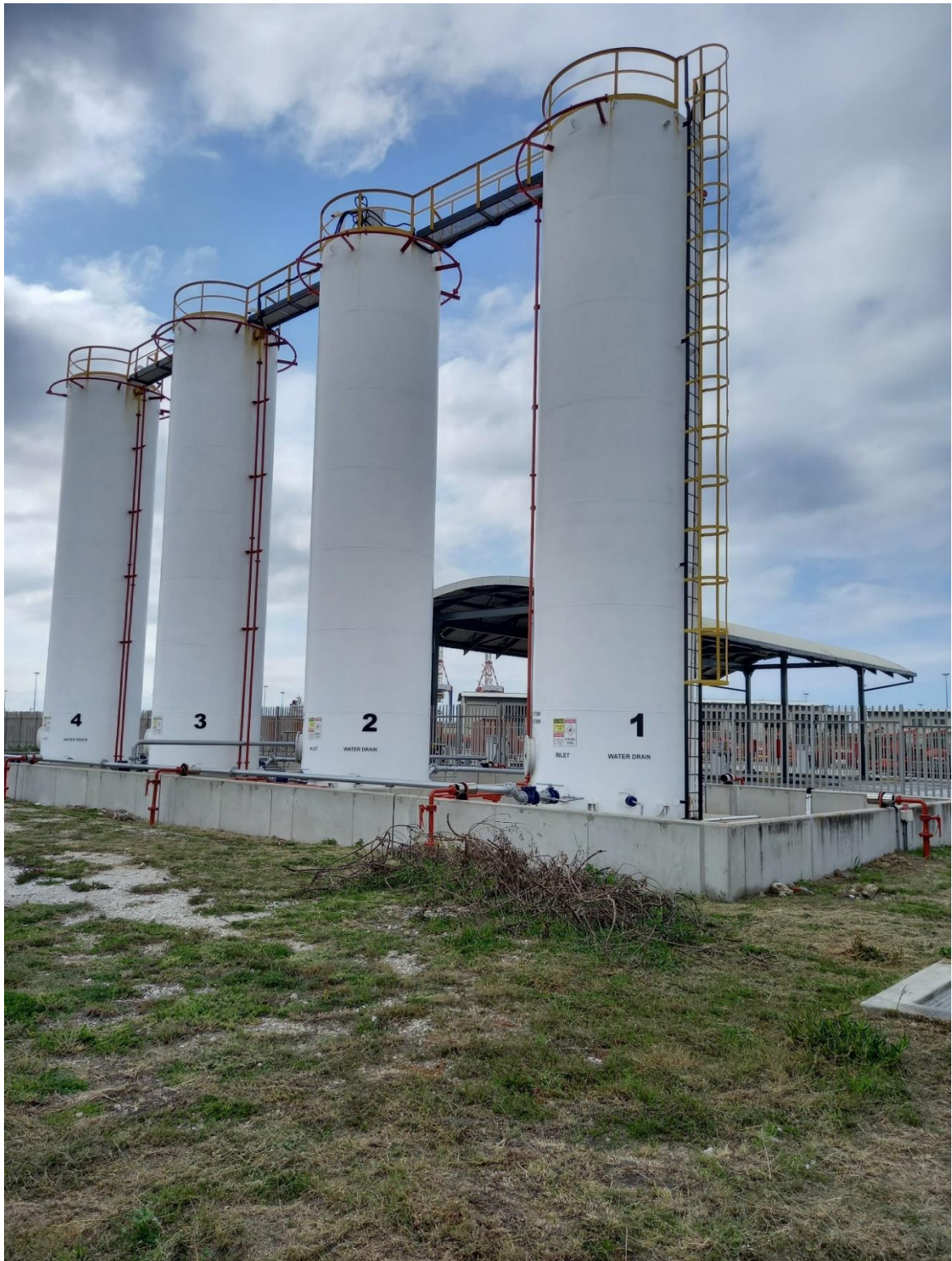
63 000 L – 4 x Diesel Tanks
