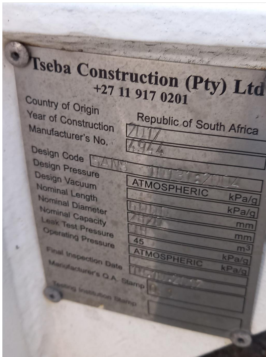
Name Plate on the Tank
