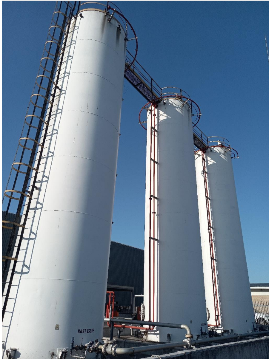
Tank Size: 915 mm diameter x 12.6 meter high: (3 Tanks)
