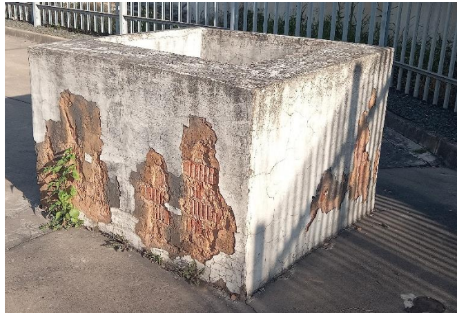
Sump Tank to be coated
