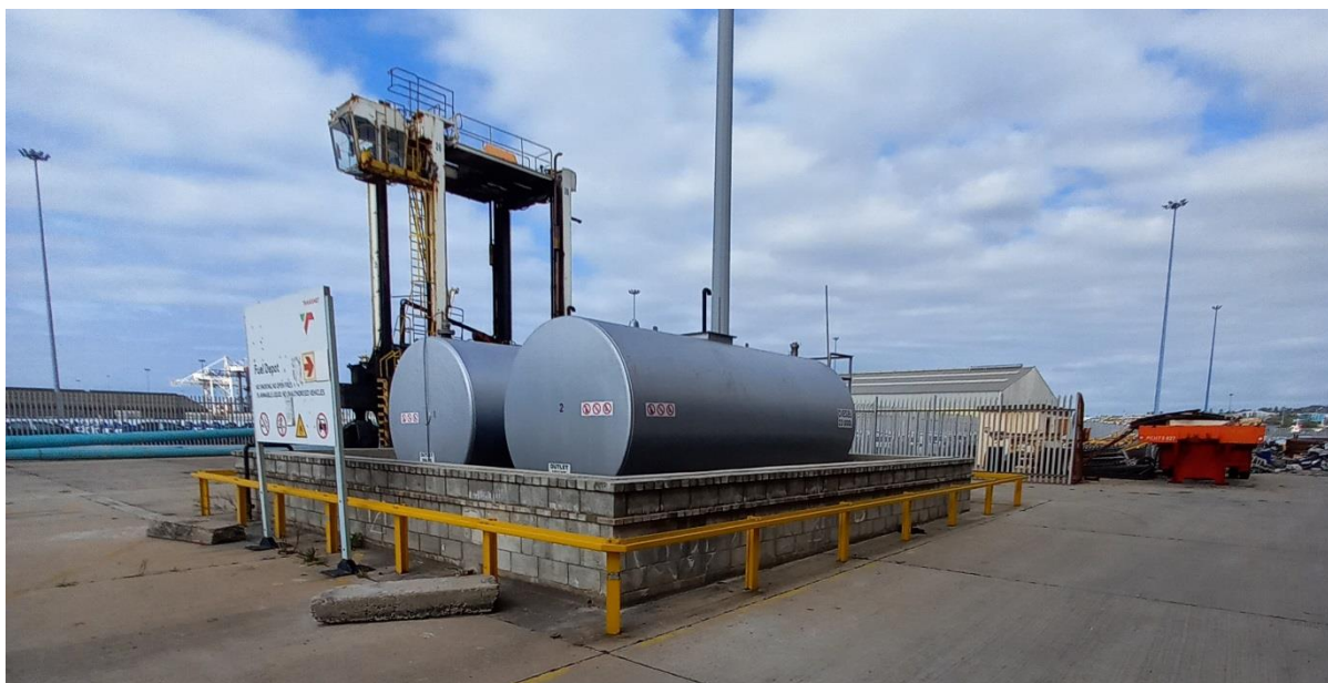
2 x 23 000 L horizontal Aboveground Tank: Diameter 2.3 m x 5.4 m Long
