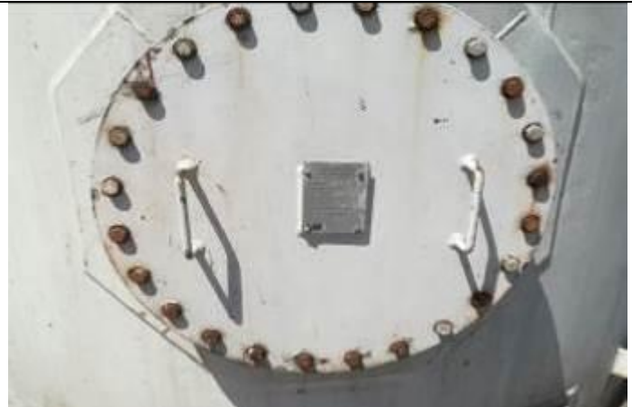
Rusted manhole bolts
