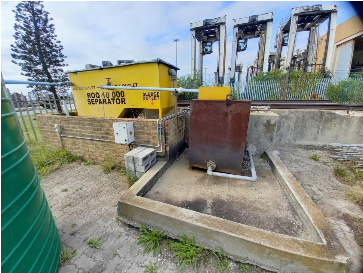
Oil spillage collection and filter area
