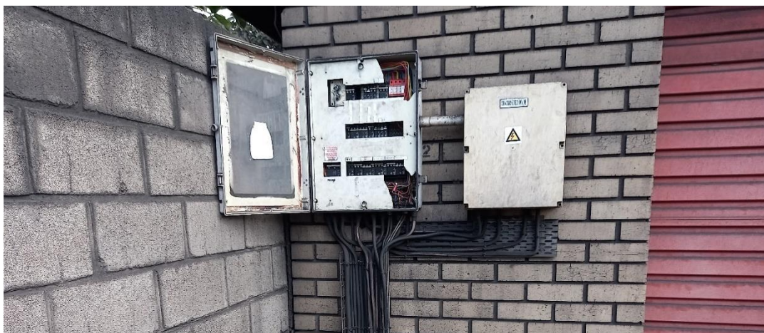
Photo of Electrical cables and the Distribution Board
