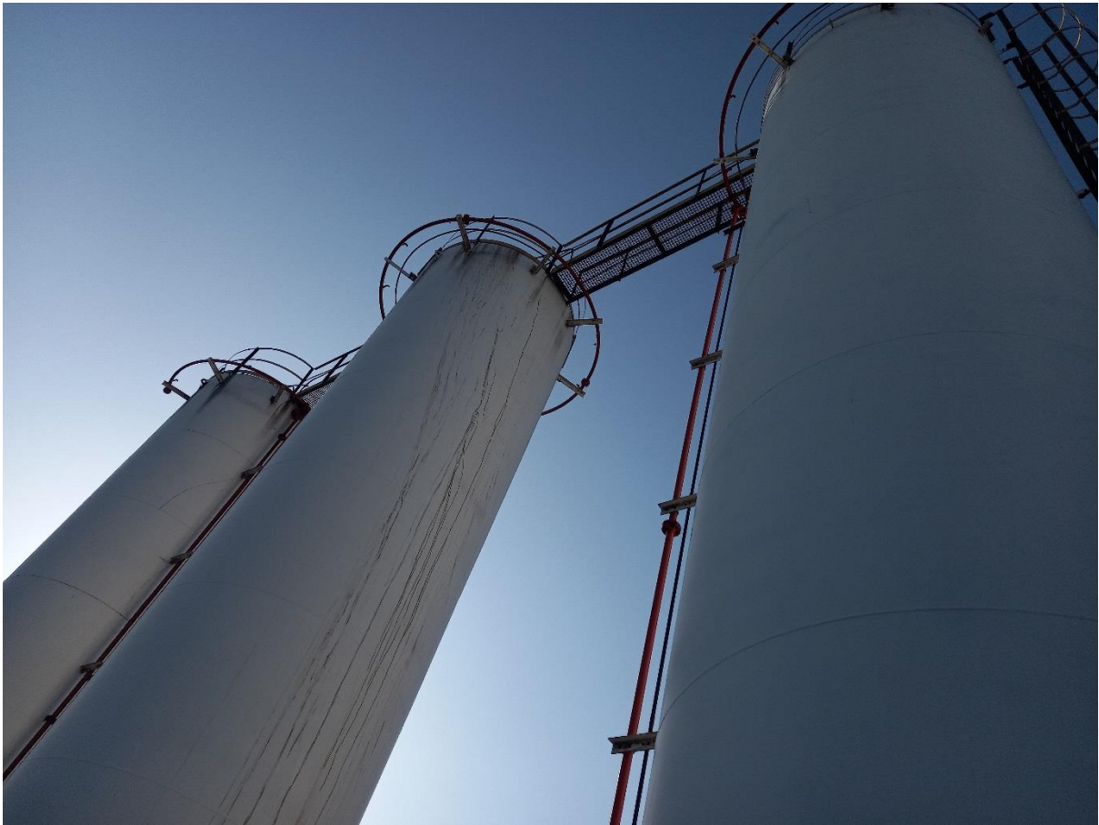
Stain on the Tank indicates that overfill system is not working
