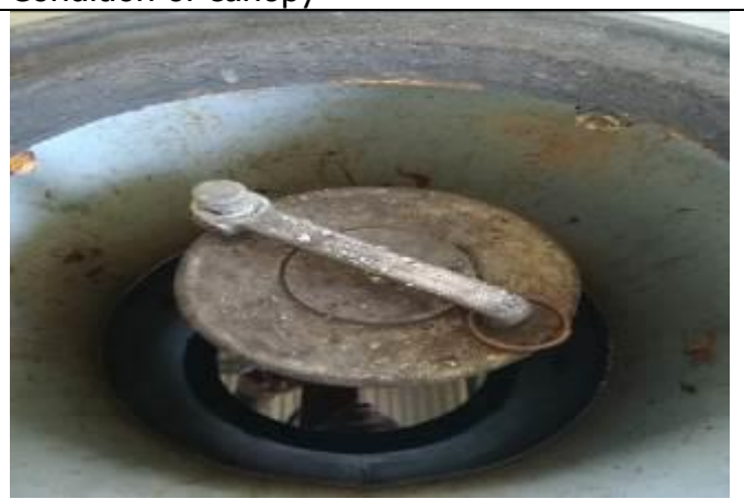
Diesel in the receiving line (Leaks)
