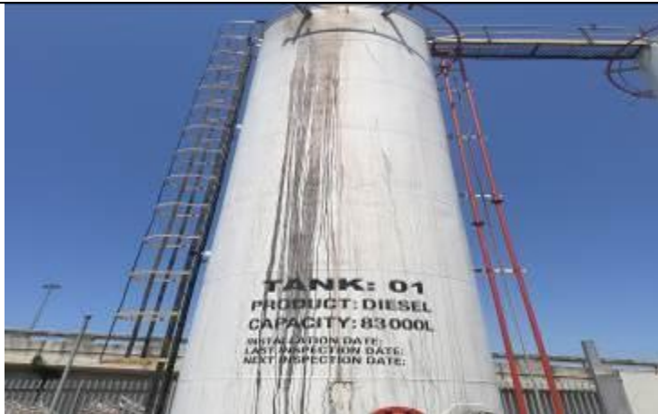
Tank 1 visible spillage
