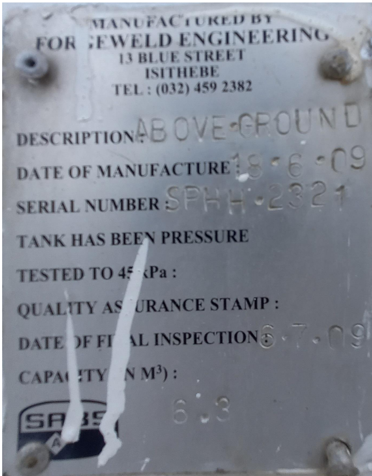
Name Plate of the Tank with 6.3 000 L Capacity
