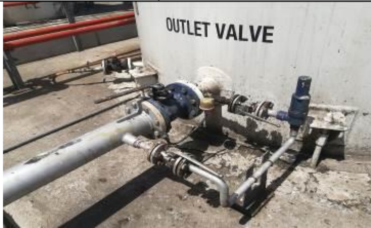
Tank thermal relief
