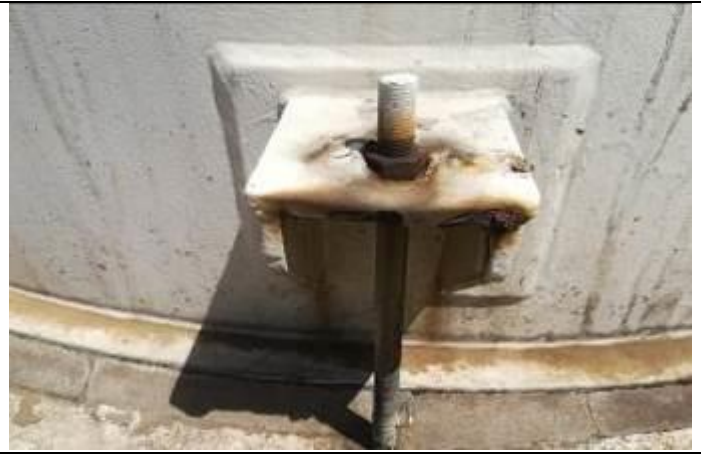
Rusted tank anchor
