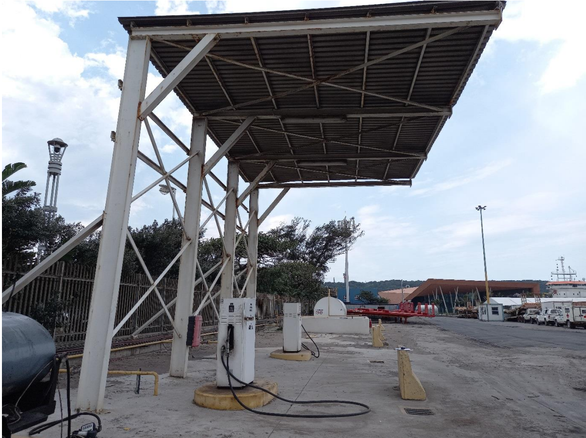
Photo of Point Road Diesel Tank and dispensers
