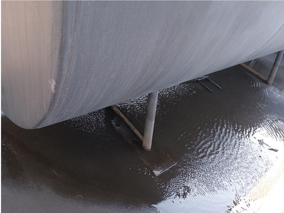
Base plate and supports are getting corroded in the storm water
