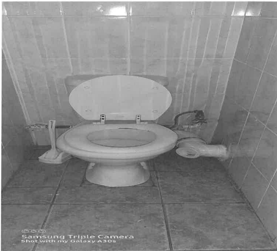
Toilet to be replaced with new, galvanised pipes to be replaced with copper pipe with new angle valve.
