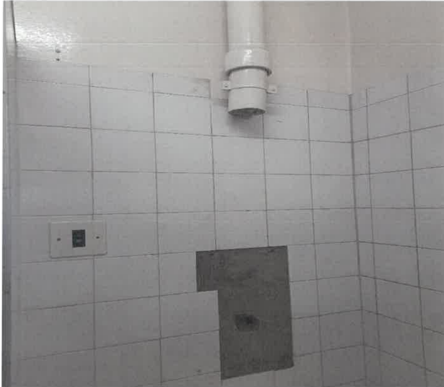
Incinerator chimney to be removed, opening to be sealed and made good.
