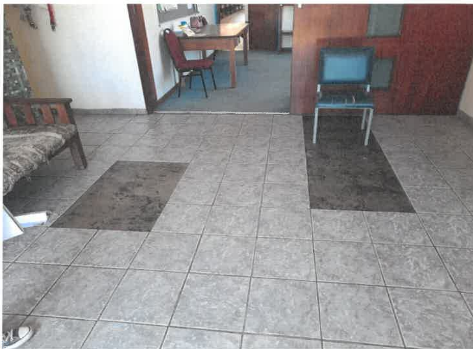
The floor tiles are broken and out, they need replacement
