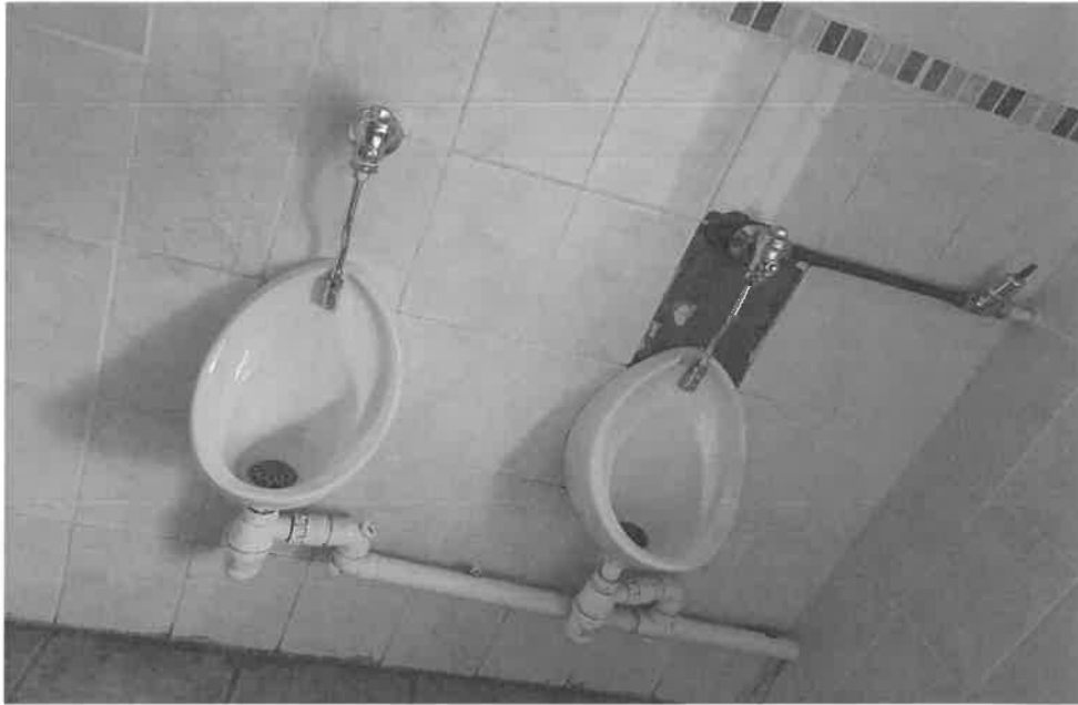
Waste pipes leaking, flush master leaking and Stopcock faulty.
