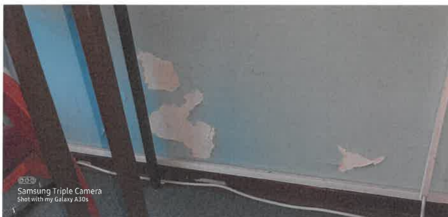
Painted surfaces to be cleaned and repainted.
