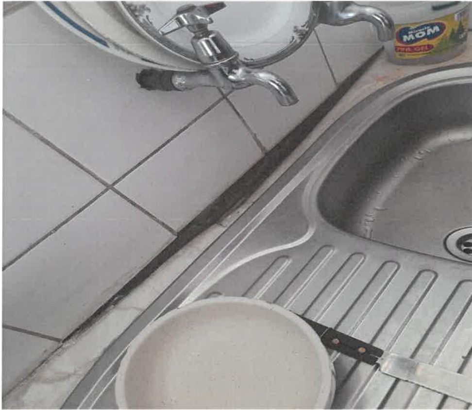
The sink taps are leaking as the results the countertop got damaged.
