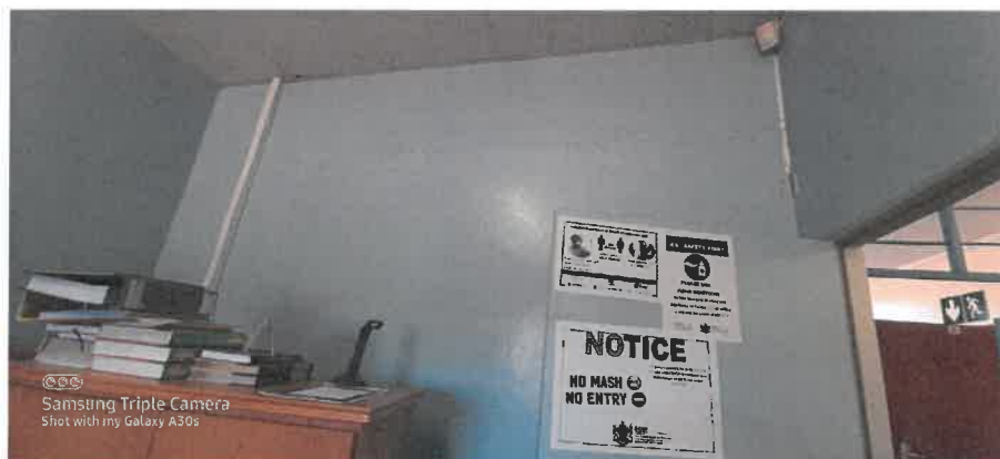
Incinerator chimney to be removed, opening to be sealed and made good.
