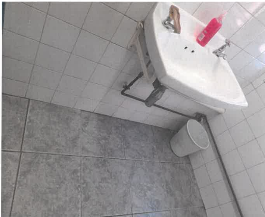
Hand wash basin to be replaced complete with waste pipes and fittings, leaking taps
