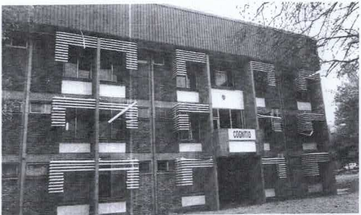
Photo 1: Front view of D4 accommodation block with indication of the levels, bottom, middle and top floor with metal mesh that is utilised as fly screens in front of windows.
