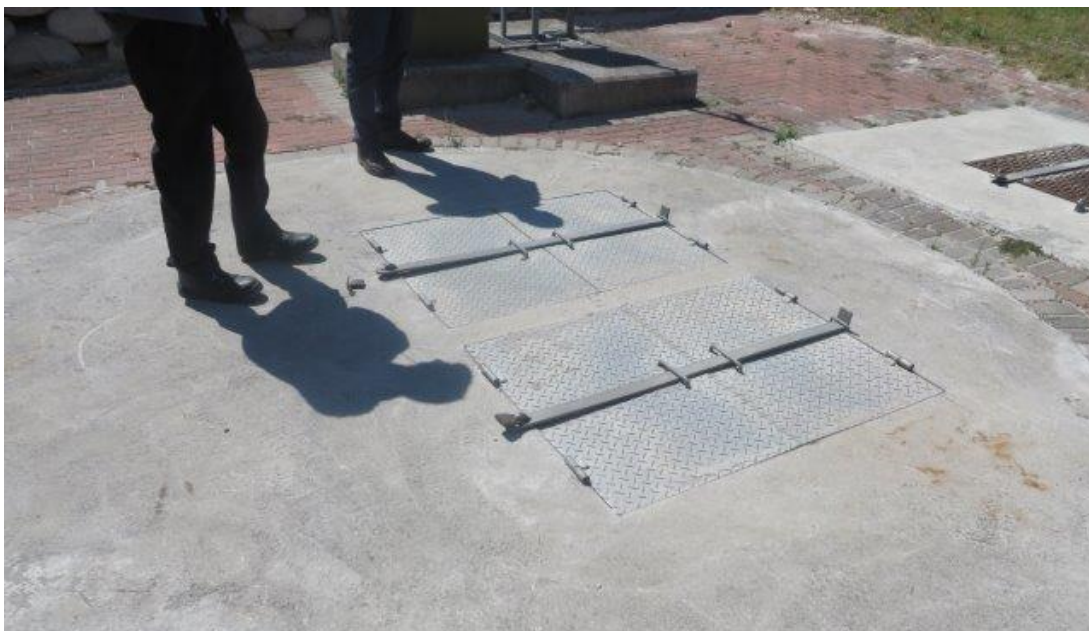
Photo 12. Stormwater sump – Freight road under pass.
