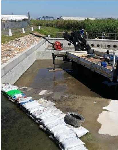
Photo 15: ACSA pond being emptied for cleaning purposes.
