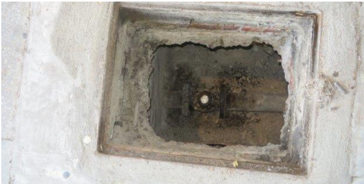
Photo 15. Damaged water meter opposite CT
