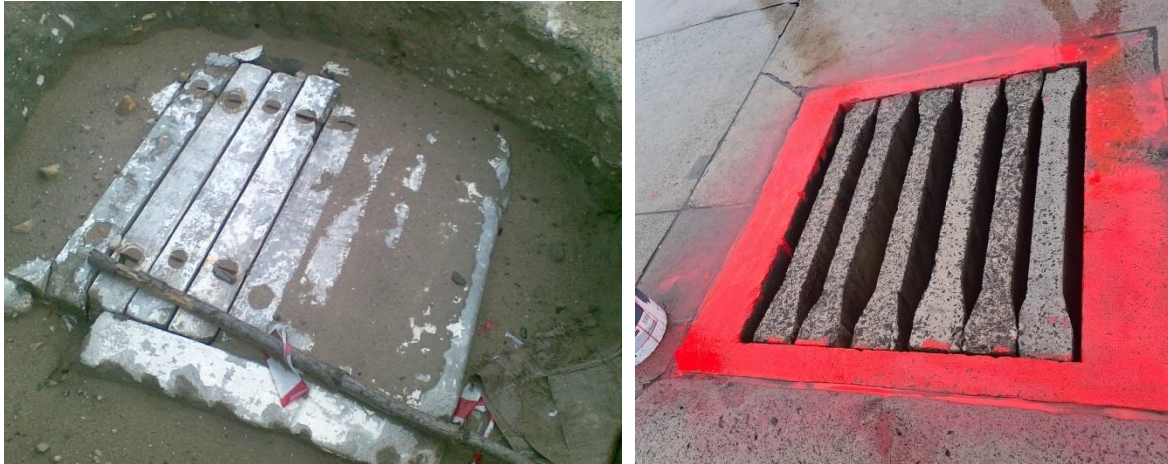
Photo 18: Various special design of manhole covers in airside (aircraft movement area)
