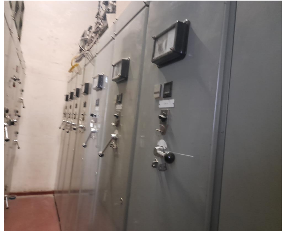
Figure 5 Old LV switchgear of fuse technology and working space
