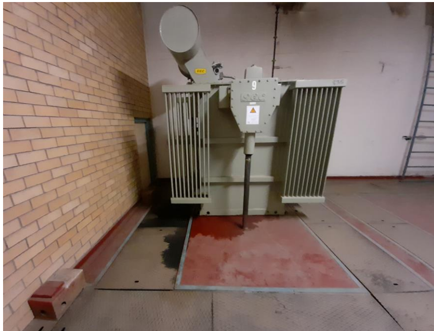
Figure 2 Distribution transformer with no oil containment provision
