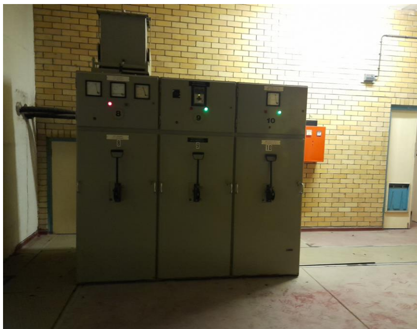
Figure 3 Medium Voltage Oil Insulated Switchgear
