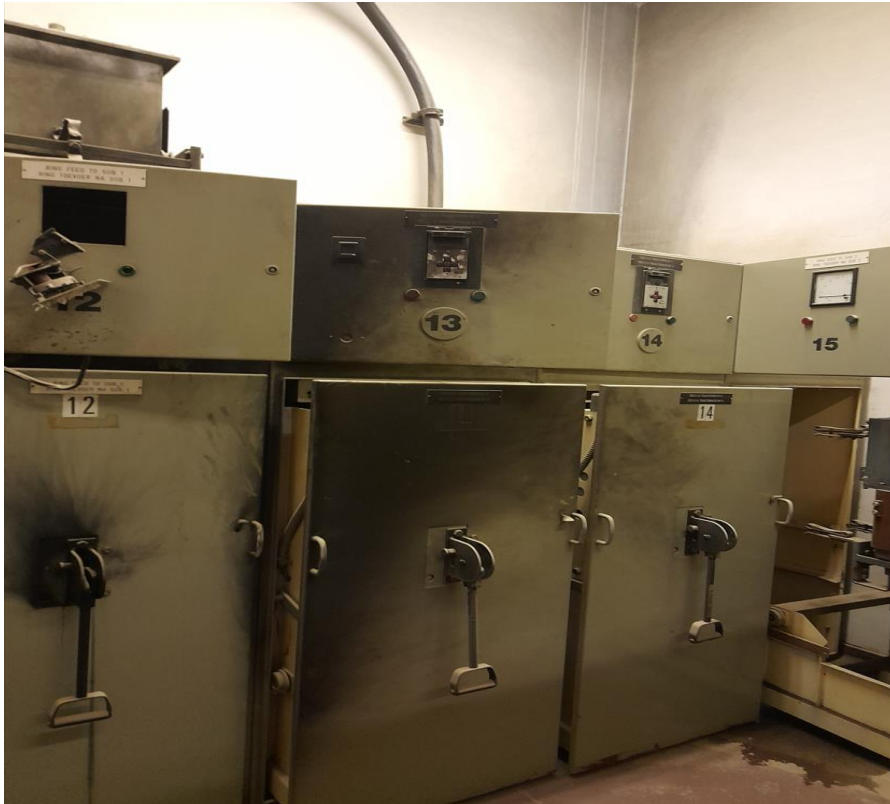
Figure 4 MV Switchgear exploded and out of service
