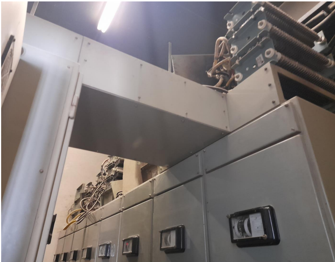
Figure 7 Old and Obsolete Resistor Starters technology
