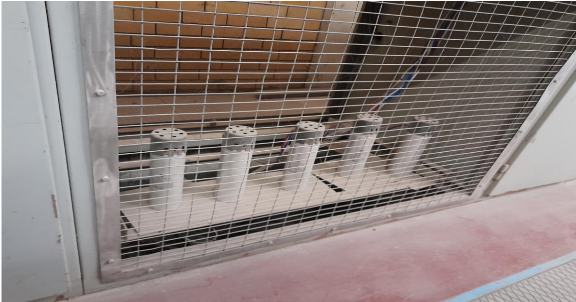
Figure 6 Old and Obsolete Power Factor Correction
