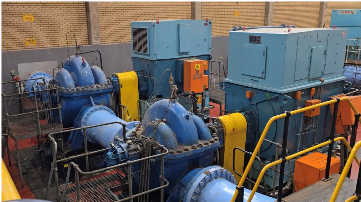
Figure 1: An image of a typical multistage MV pump-set.
