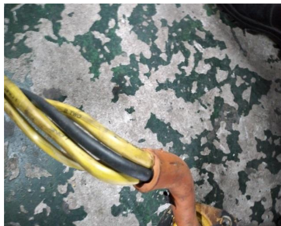
Fig 1 – two core, 25 mm 2 electric cable
