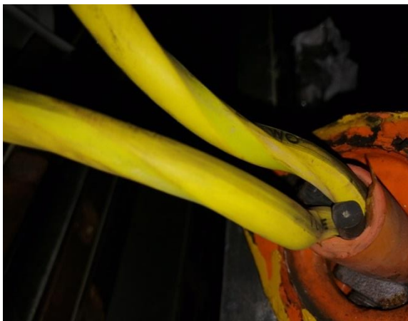
Fig 1 – two core, 25 mm 2 electric cable
