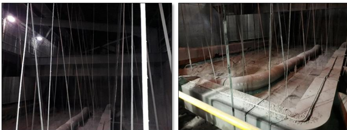
Figure 2: Wire hangers supporting the suspended ceiling
