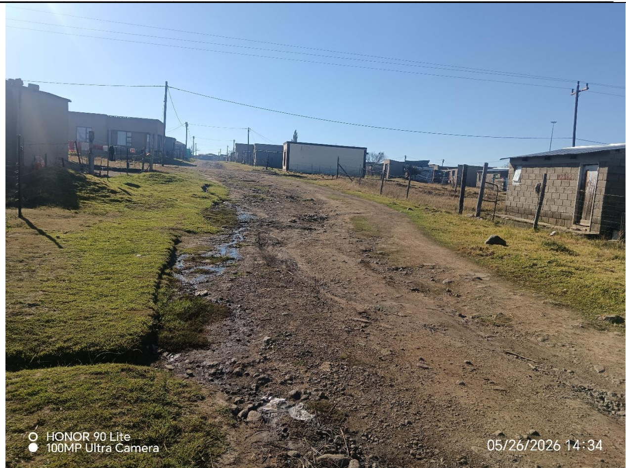
Road 1 Ward 7: Flowing water from household taps
