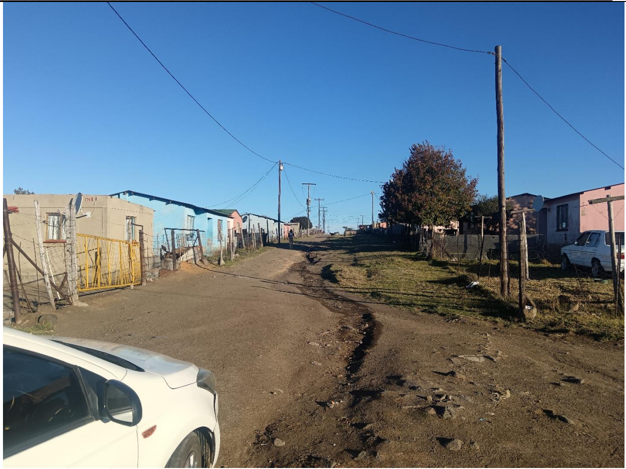
Road 4 Wrad 7: Erosion due to uncontrolled stormwater
