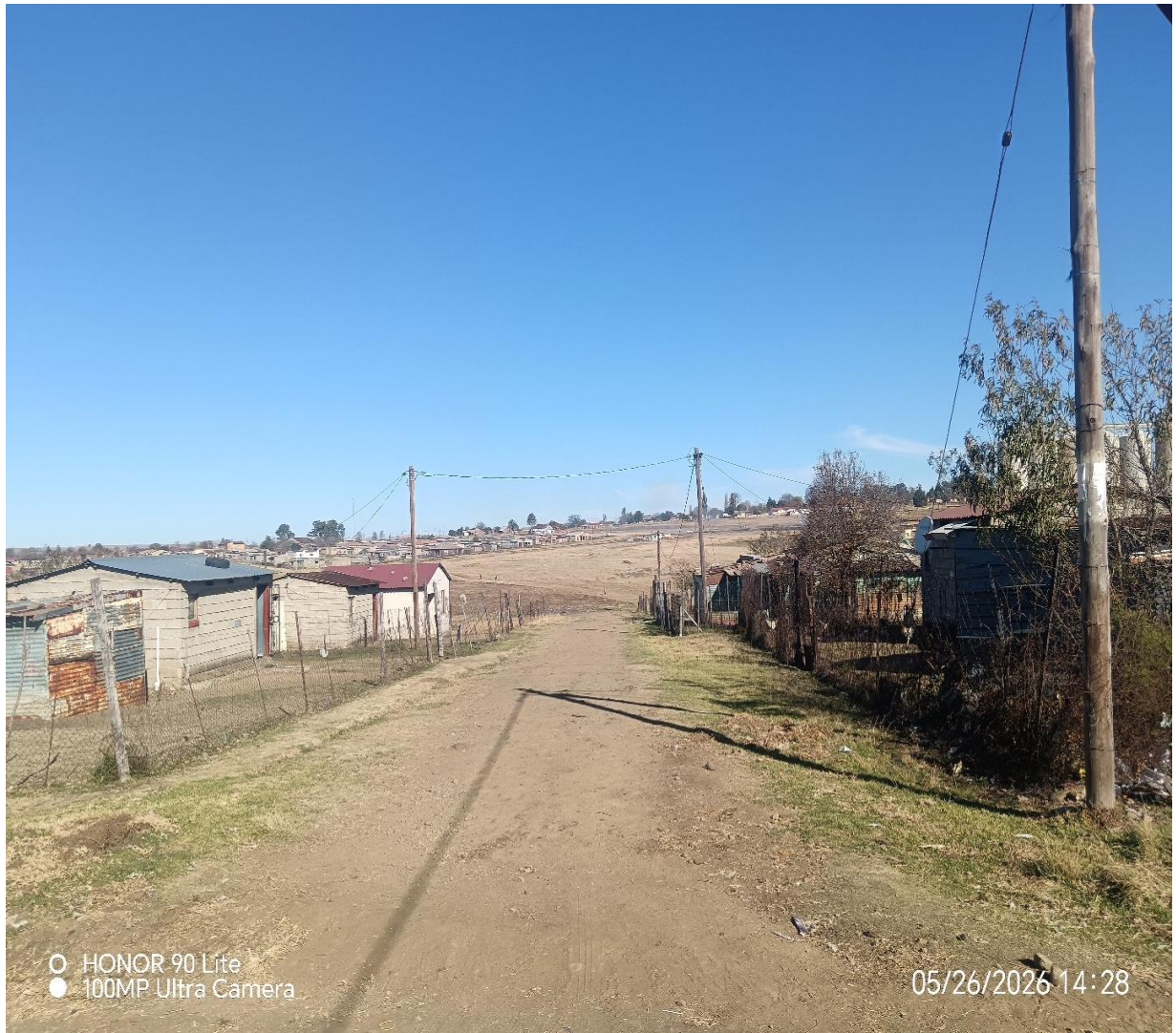
Start of Road 1
