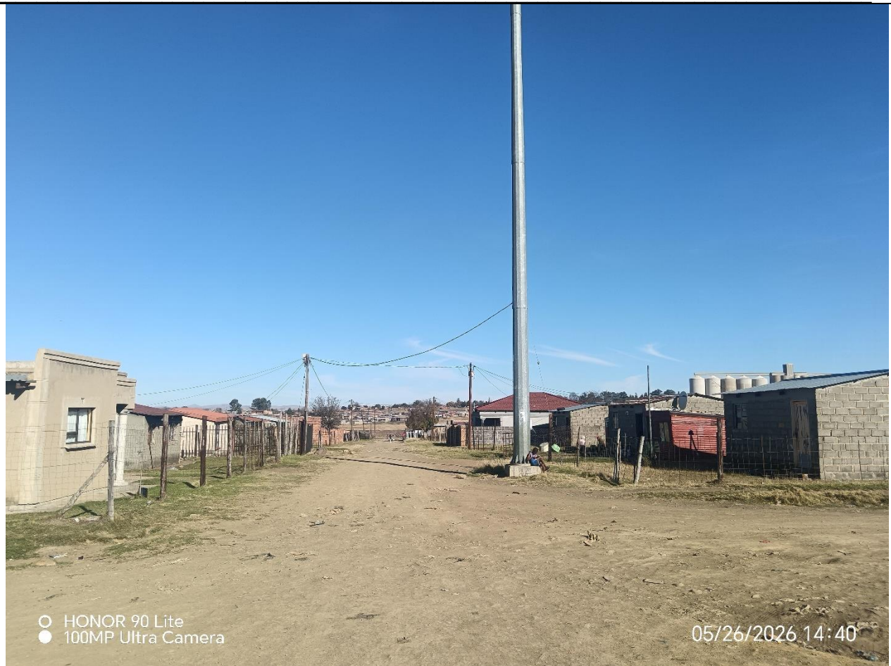
End of road 2 Ward 7
