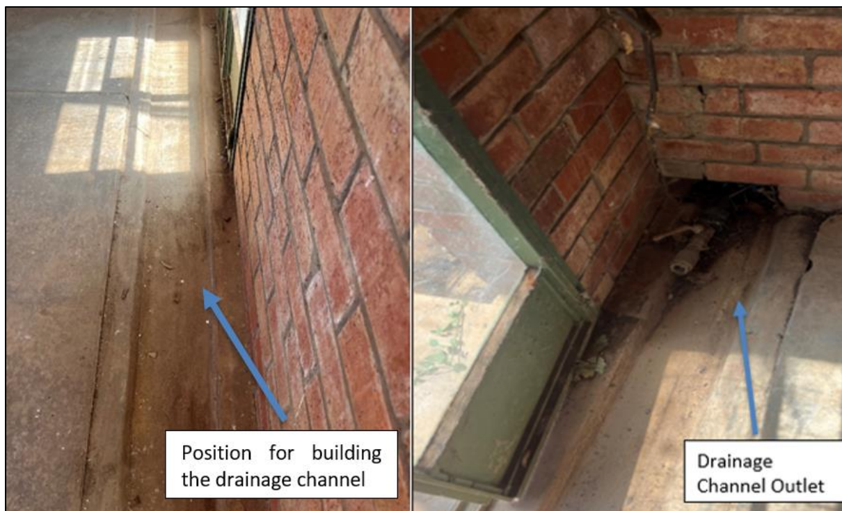
FIGURE 2-4: EXISTING DRAINAGE CHANNEL
