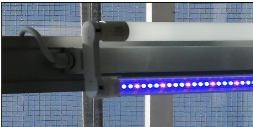
FIGURE 3-1: EXAMPLE OF GROW LIGHTS (NOTE: THIS EXAMPLE IS NOT IP65 RATED)
