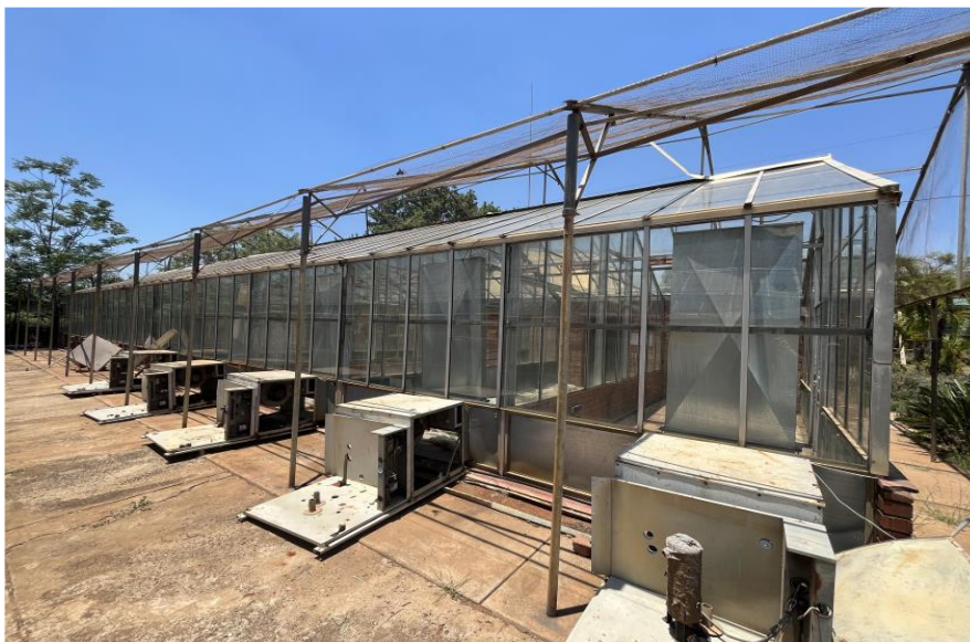
FIGURE 2-1:SIDE VIEW OF THE CURRENT B5 GREENHOUSE
