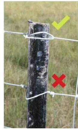
FIGURE 1: CORRECT WIRE FIXING
