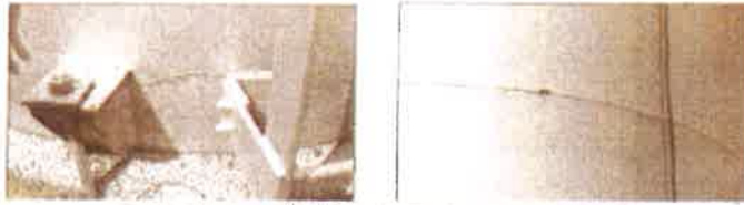
Coating failure with subsequent minor corrosion noted on tank shell
