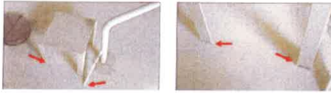
Supports welded directly to tank floor
