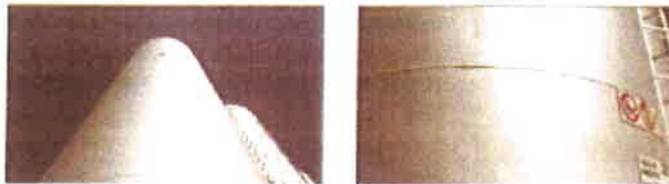
Coating failure with subsequent minor corrosion noted on tank shell
